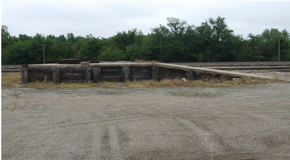
3. The loading dock at Burlingame, Kansas, looking east. May, 2008. Photo by Jared Harper
