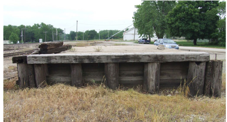
5. The platform end of the dock, looking south. Note the heavy timbers used as a top chord, and also where they are missing on the dock's sides. Also notice the heavy round poles used to support the structure. May, 2008. Photo by Jared Harper
