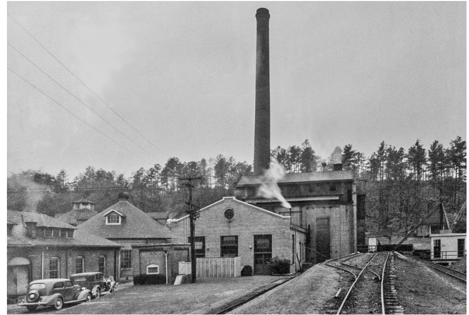
9. A view of the plant showing the tracks for the coal dump and those leading to the ash tunnel. Phillip Griffith Collection
