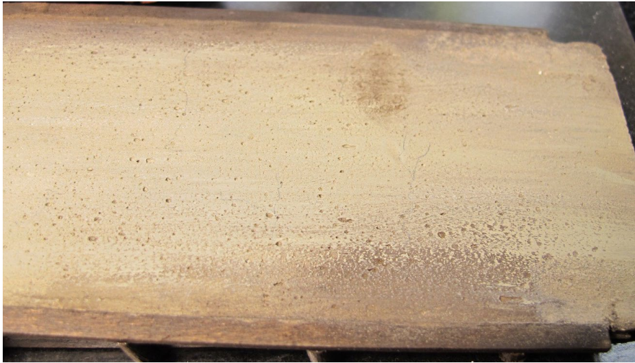
20. Top view of the ramp after weathering. Note that the wood frame on top is also weathered heavily, but provides just enough contrast in color and texture.
