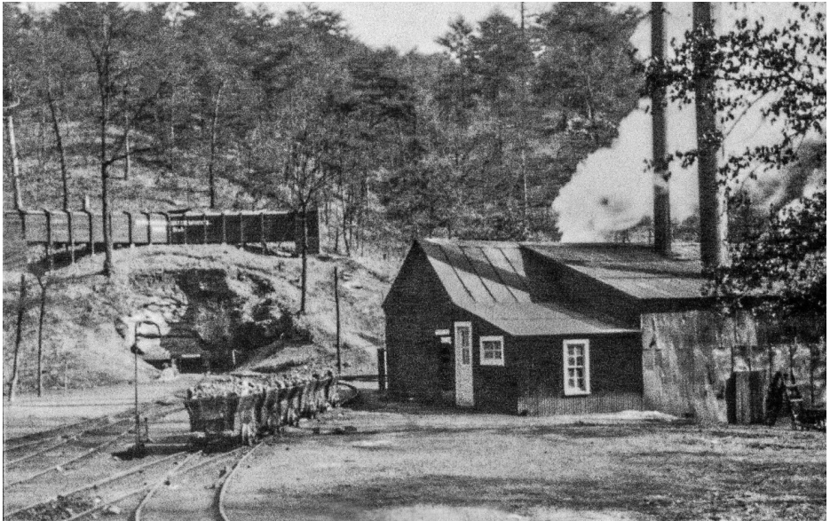
4. The Merkle Mine showing the trackage and the hoist house. The entrance can be seen to the left of the tiny mine cars. Phillip Griffith Collection
