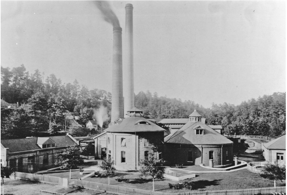
2. The Cahaba River Pumping Station of the Birmingham Water Works. Larry Smith Collection
