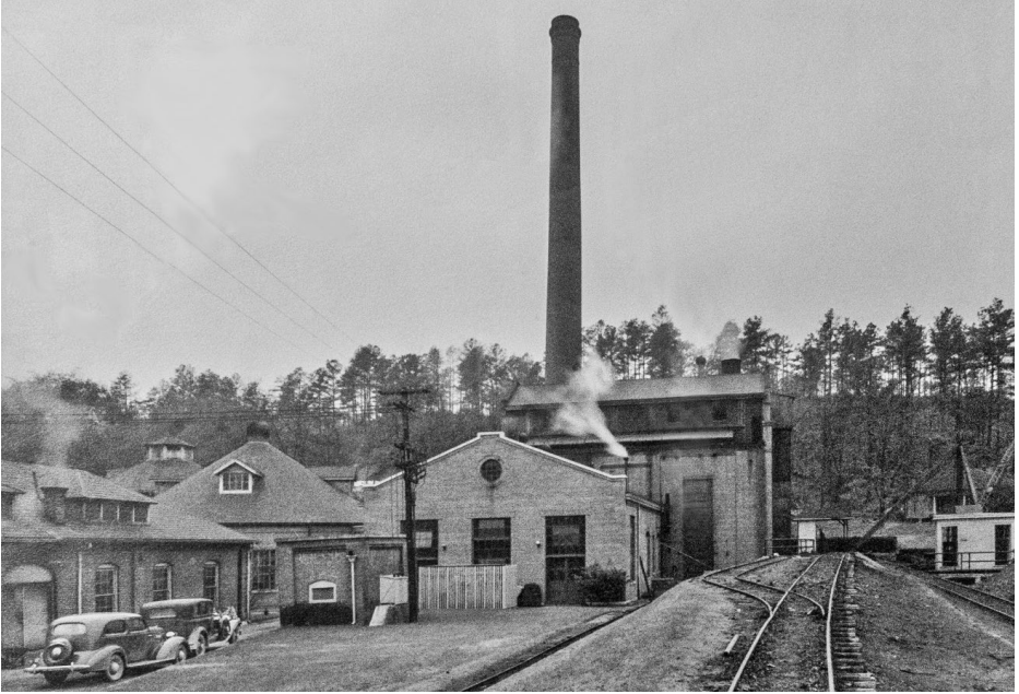
9. A view of the plant showing the tracks for the coal dump and those leading to the ash tunnel. Phillip Griffith Collection
