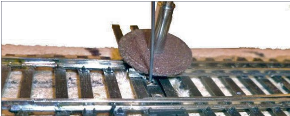
22. Cutting off the excess.
