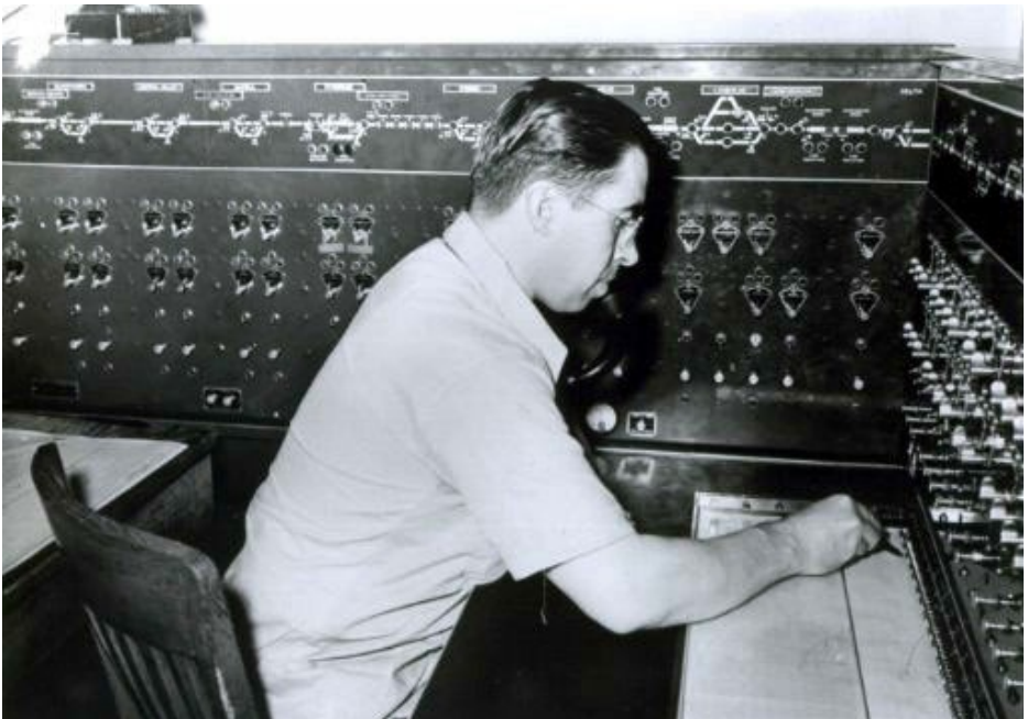
3. SP's Canyon Dispatch machine in the day. Photo courtesy Bob Jacobsen
