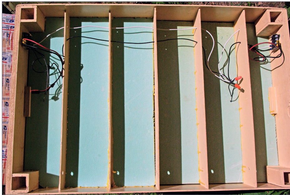
5. Polyurethane glue works excellently for bonding the foam to the painted wood, and for laminating layers of foam.
