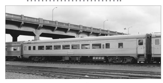
17. Chair car in the later lettering for Overland service, car 2432 in class 77-C-3. The drop-equalizer type trucks are replacements, usually taken from a scrapped sleeping car The car still has its original fluted sides. *Courtesy Bob's Photos*
