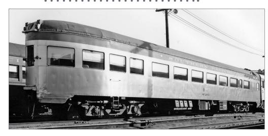
19. Parlor car 2951, class 77-PRO-1 parlor observation in its final configuration shown in San Francisco as of April 1971. The car has late box type rear lighting array, flat stainless steel sides with red letterboard stripe, and Waukesha air conditioning. Propane bottle containers show under the car. This car still has its triple bolster trucks.
