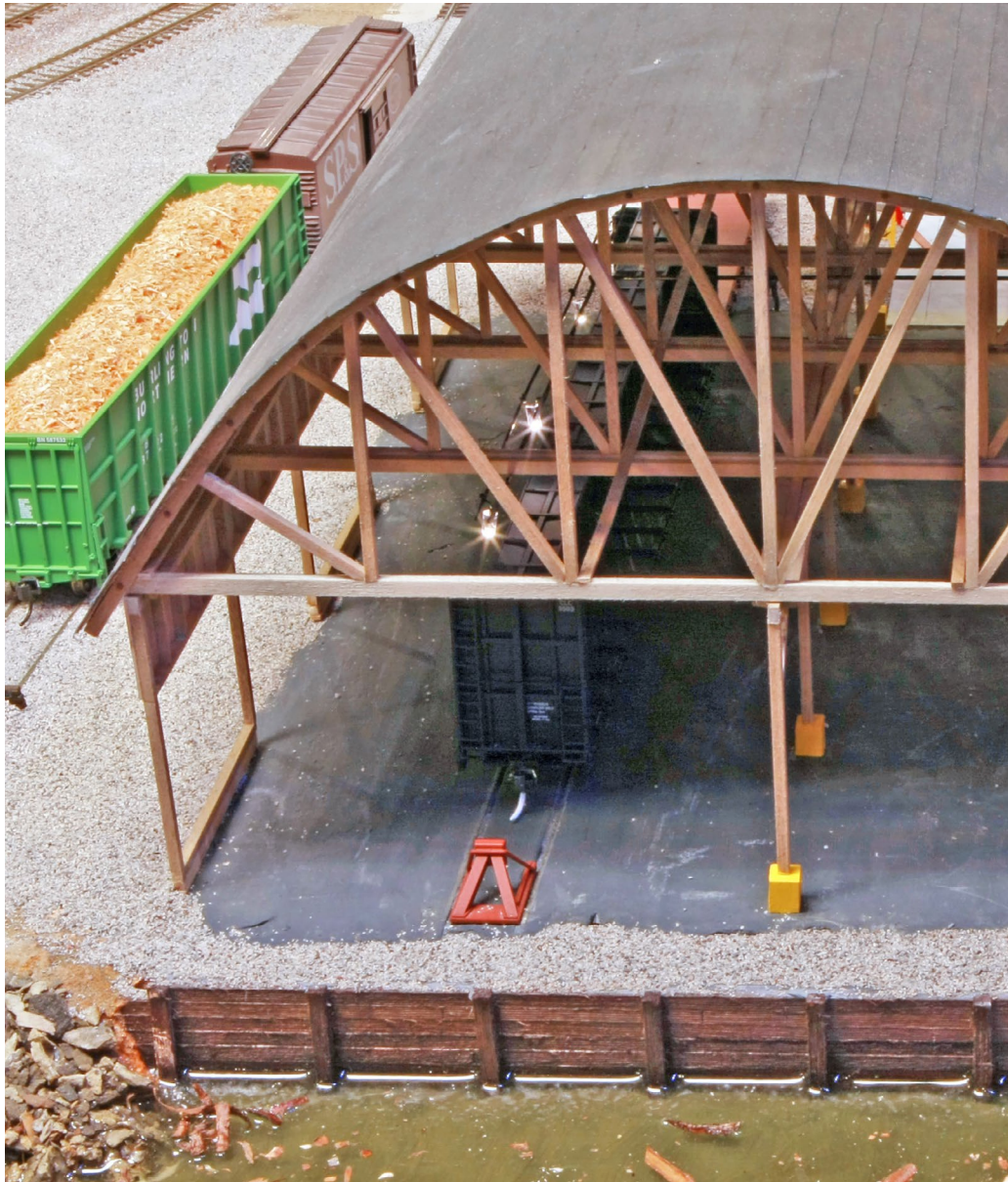
11. Next, is this close-up of the lumber mill's curved-roof loading area. This curved truss roof construction was quite common for lumber mills located in the Pacific Northwest.
