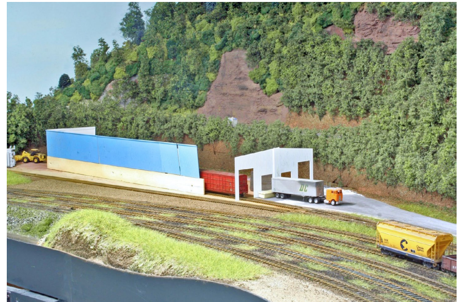
2. Panels from Pikestuff and Walthers are mocked up on the layout site before the Masonite building construction starts.
