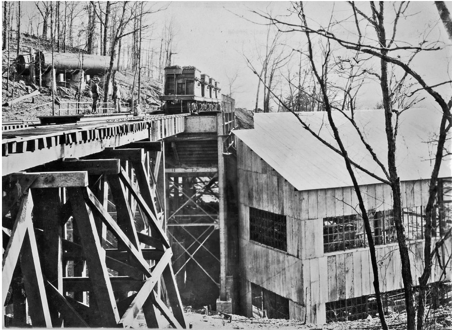
14. This “high line” apparently ran from the surface mine operation to the washer, which was under construction at the Vance Mine in the winter-spring of 1928-1929. John Stewart Collection
