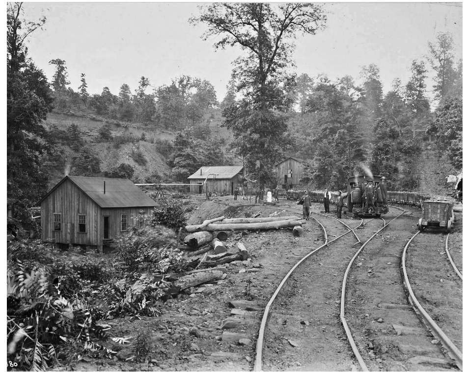
9. Hoist house and narrow gauge at the #2 red ore mine. John Stewart Collection
