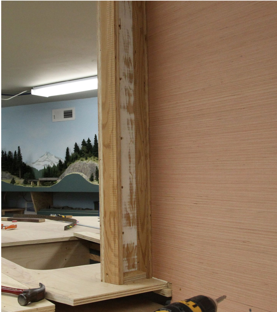
4. Here's an inside view of the bullnose's mounting plate. It's made of three pieces of plywood and is attached to the benchwork and the backdrop support cleat in the ceiling. I used my trusty copy of 3rd PlanIt layout-design software to figure distances and angles (5). The backdrop plywood separates about 24" from the end of the backdrop and each piece is screwed to the mounting plate, holding it firmly in place.
