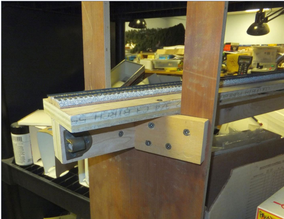
36. The catch is on the land side of the bridge. Supporting pieces are all screwed in place with high quality square-drive screws.
