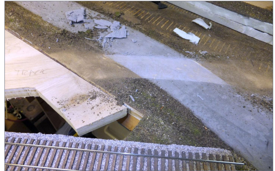
29. To prepare for laying the bridge track, I removed all of the scenic material to permit the track to lay perfectly flat coming off the bridge. My staging area is all Custom Trax. The product is no longer available – real wood ties glued to high quality cork roadbed, and ballasted and weathered with code 83 rail spiked in place with a Kadee spiker – so I wanted to use a few leftover pieces to continue the track out of staging and across the bridge.
