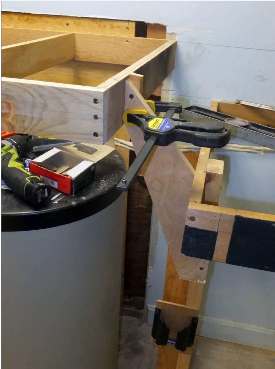
11. Sometimes a piece of plywood needs to be custom-cut to connect different levels.
