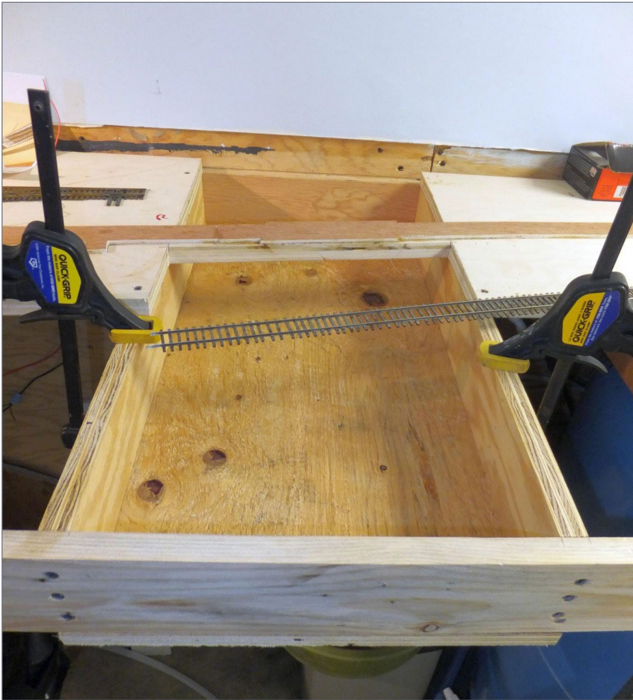
44. The base for Tunkhannock Creek has a plywood floor to support the creek bed and bridge abutments.
