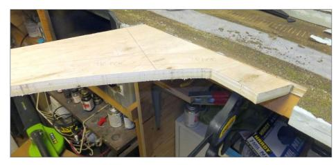
28. The new sub-roadbed is now continuous from staging across the aisle onto the layout in the distance. Note that the bridge hinge and latch points have not been cut at this time.
