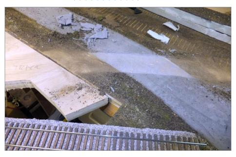
29. To prepare for laying the bridge track, I removed all of the scenic material to permit the track to lay perfectly flat coming off the bridge. My staging area is all Custom Trax. The product is no longer available – real wood ties glued to high quality cork roadbed, and ballasted and weathered with code 83 rail spiked in place with a Kadee spiker – so I wanted to use a few leftover pieces to continue the track out of staging and across the bridge.
