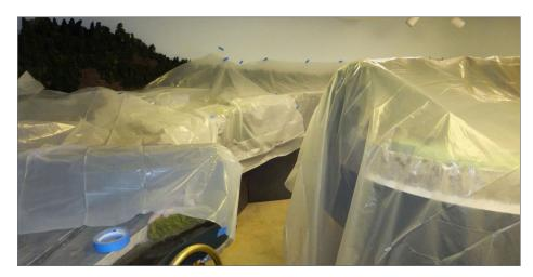
3. The tarps were an excellent idea! They were removed very carefully after I used the vac with a brush attachment to get most of the fine dust off.
