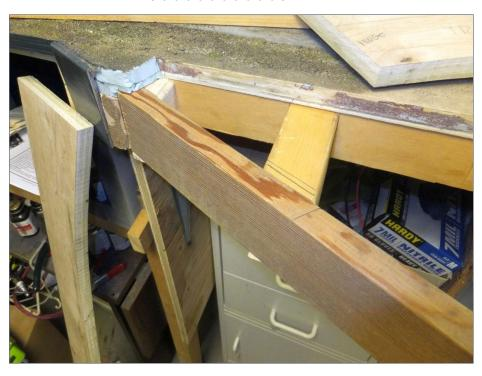
31. Next, I used a nice piece of vertical grain fir to form the attachment point. This type of fir has the smallest chance of warping of any wood I know.
