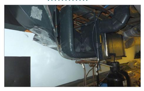
2. The air handler, water filters and associated piping. What's not to like?
