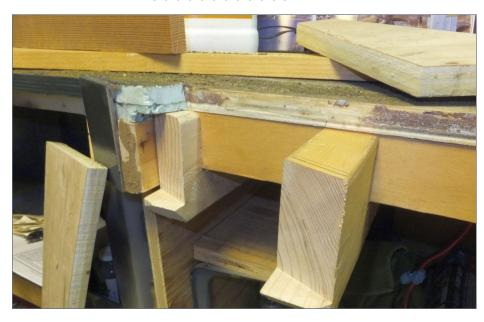
30. My first step in creating the bridge footings was to make a couple of pieces using 2x6 material that would have the correct orientation to the bridge hinge, and also be firmly attached to the existing benchwork. I notched them around the existing 3/4" deep plywood supporting the plywood on top of the layout, and screwed them to that as well as to the support member.
