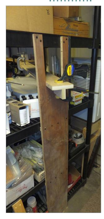
34. On the latch side of the bridge, I needed a very solid support and plastic shelving would not work. I chose to add a piece of supporting plywood, notched as shown. mounted on the concrete floor, and screwed to each shelf on the way up. The plywood sub-roadbed going back into staging has a hefty "T" support.
