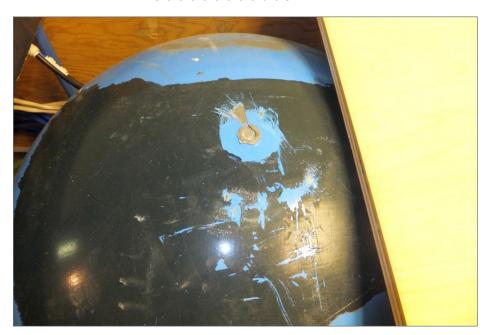
16. My friend Dave was alarmed when I took a Sawzall to the top of the Welltrol! I called the company on the phone to ask about this nut. It's used in the manufacturing process to allow them to transport the tank during construction and painting. Ask before you saw!
