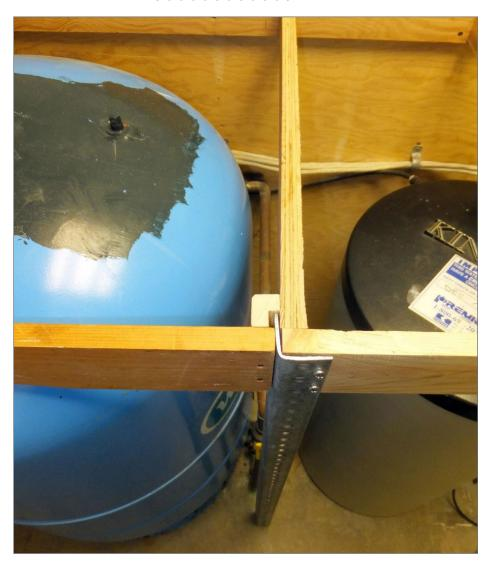
15. The pre-punched metal angle iron (one on each side of the Welltrol cylinder) proved to be a perfect small footprint support leg for the new bench work. I made a custom mounting bracket out of wood for the removable front piece. The bracket wrapped around each metal support leg on the left and right of the cylinder.
