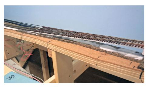
47. Caulk was applied to the cork roadbed under the turnout and the turnout set in place.
