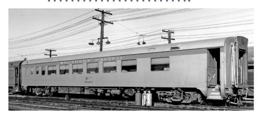
10. Prototype chair car 2354 in class 83-C-5 built in 1954 of steel for the Coast Daylight. *Courtesy Bob's Photos*
