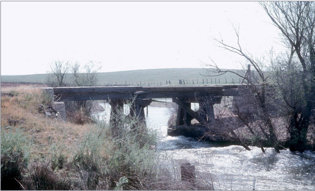
4. This photo of the remains of the trestle over Edendale Creek was taken in the late 1970s, long after the rails had been removed. The bridge itself is now gone.
