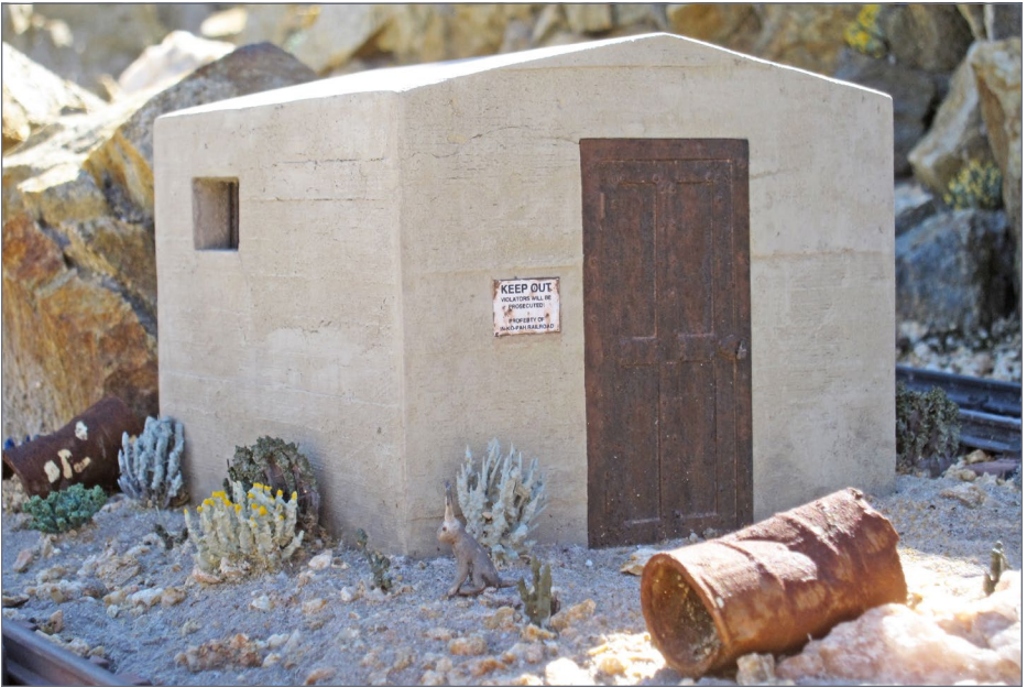
6. A former jail, this cast concrete building now provides storage for the railroad.
