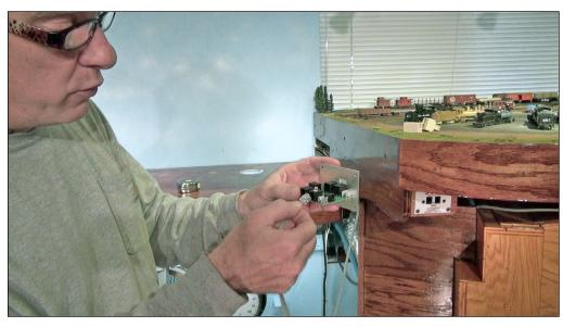
7. Then, place this wire in the jack on the back of the LocoNet panel. The wire is measured and cut to fit into the next panel, where you will install another phone jack connector, and so forth all the way around the layout.
