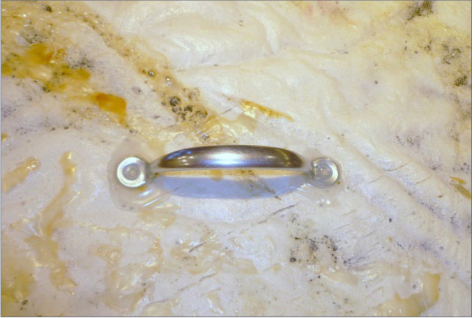
83. Handle on the bottom side of the hatch.
