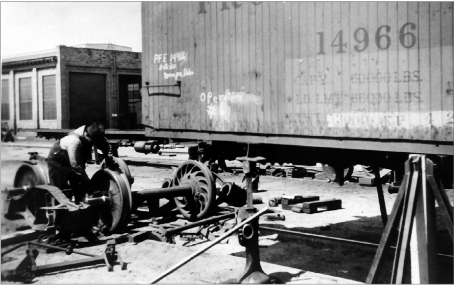
32. Same scene as previous page, at Nampa Shop, with the truck now disassembled and the wheelset ready to remove. Pacific Fruit Express photo, Milton G. Sorenson collection
