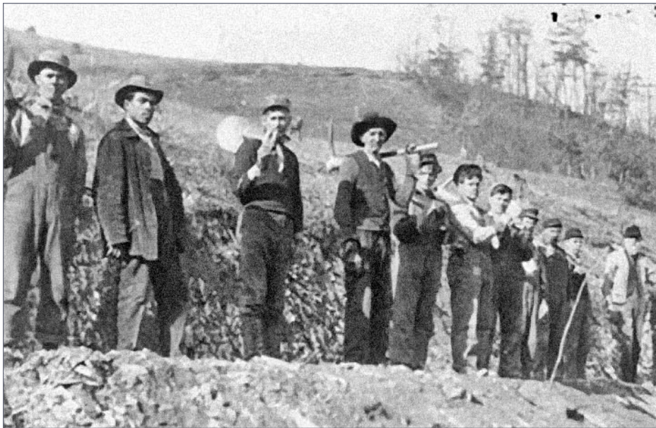
2. Construction of trestles on the TM&P and workers. From the internet, source unknown.
