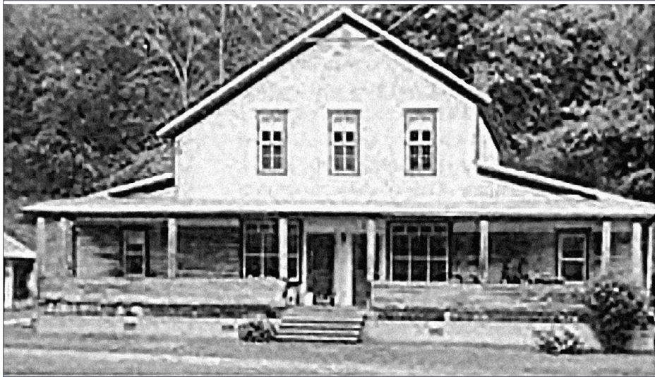
13. Russelldale station as restored to a private residence in 1993. Photo courtesy of Patricia and Charles Bonar, Larry Smith collection
