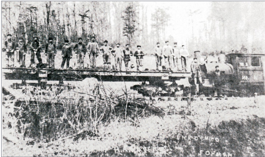
1. Construction train on the TM&P showing the 0-4-0 Potomac Construction locomotive #1. The "dinky" and crew were photographed between Barksdale and high trestle. Note the homemade number on the locomotive. Philip Miltenberger collection, published in the March 1987 Light Iron and Short Ties
