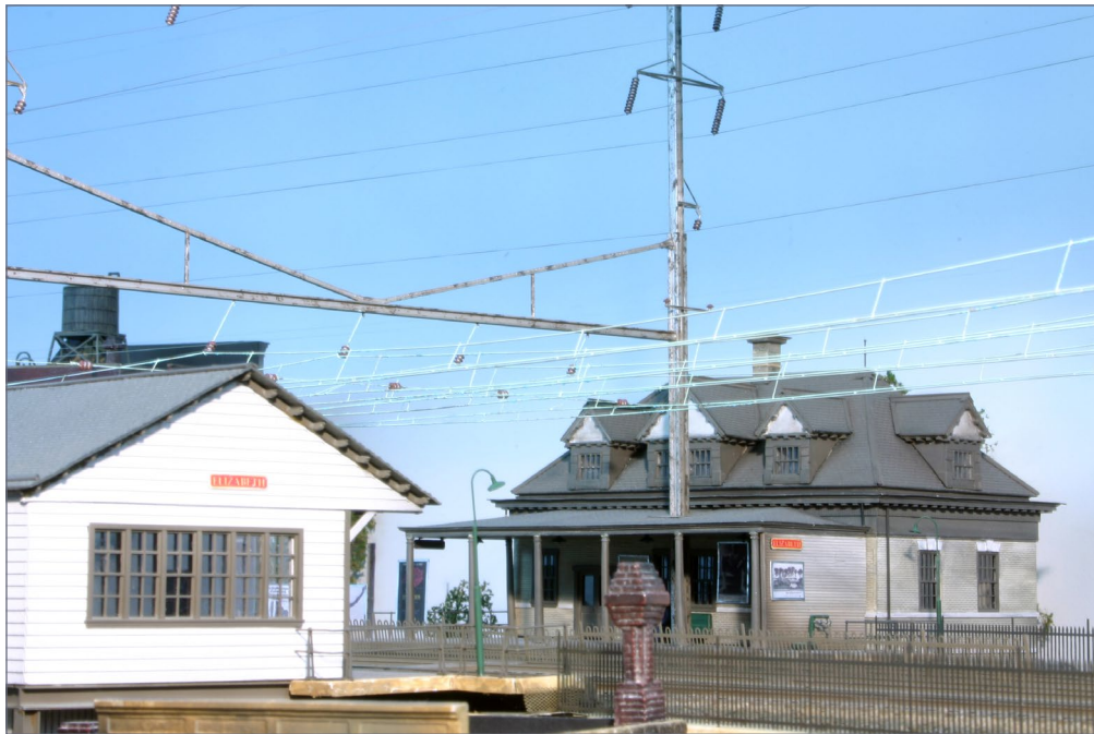
25. Andy scratchbuilt the station and waiting room at Elizabeth from styrene strip and sheet to match the prototypes, but he did compress them slightly to fit the scene.
