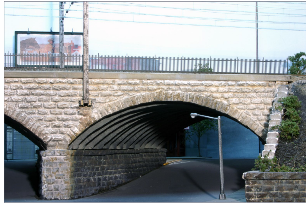
18. Andy made the twin arch bridge over North Broad Street from a modified Model Railroad StoneWorks cast plaster kit. These two arches were sandblasted clean (presumably as part of a downtown sprucing up project) in the spring of 1967. That’s why the twin arch is a lighter color than the others. The cigarette ad on the billboard also dates the scene.
