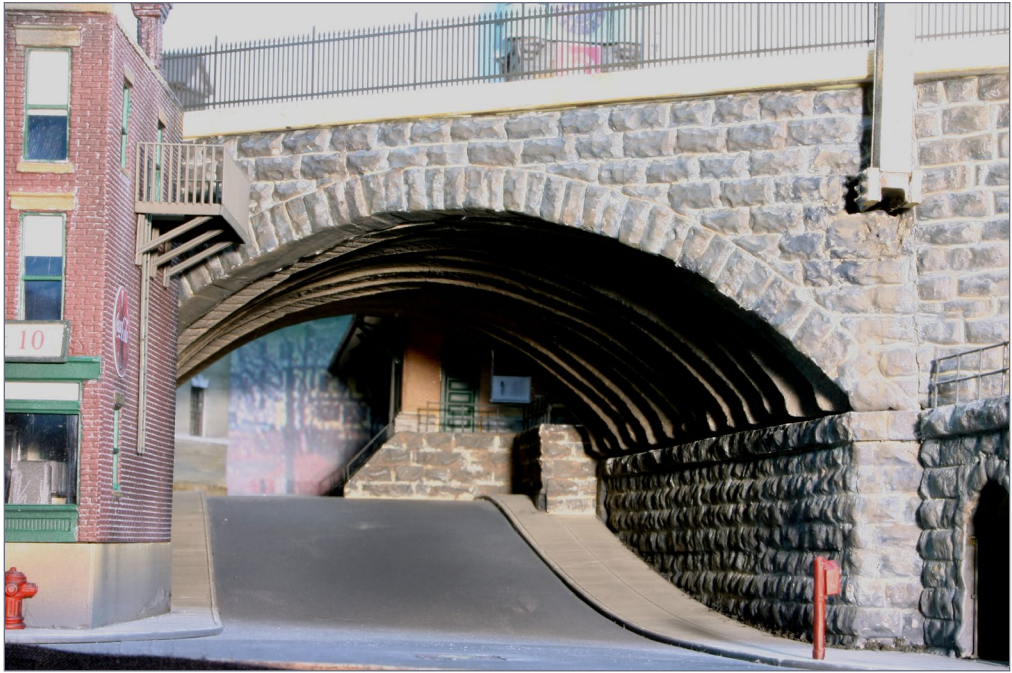
29. The angled twin arch viaduct over Broad and Jersey streets is one of several signature scenes that define the area as Elizabeth on Andy's Pennsylvania Railroad.
