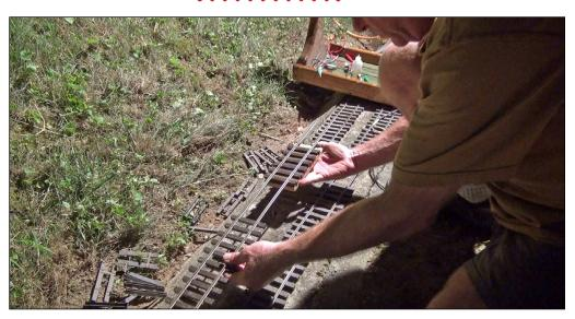
2. This process included replacing some damaged plastic ties with fresh new ones. With the help of a handmade wooden jig, the ties slide on to the rails.
