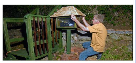
9. I built a waterproof box of wood on a pole, with a hip roof, to house the electronics and power supply. This was hidden under the deck before but I erected it on a pole for better radio reception with the hand-held radio controller.
