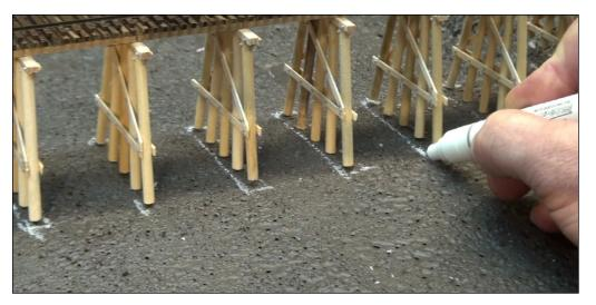
38. I placed the bridge on the diorama and used a white marker to show where the bents would be sunk into the foam scene. I then cut these grooves out with a Dremel motor tool and a router bit attachment.
