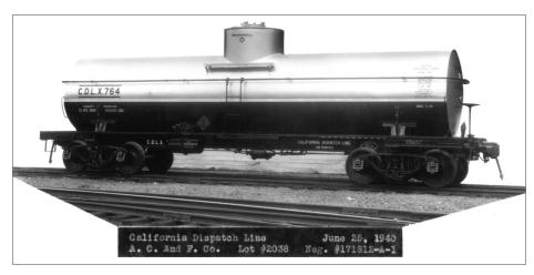
7. A California Dispatch Line insulated tank car, built for wine service, with National B-1 trucks. AC&F photo, courtesu Fd Kaminski
