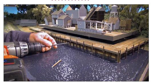
9. Using a 10-inch-long 3/16 bit, I drilled horizontally through the foam under the dock, creating a channel to run wires. I pushed a 1/8-inch diameter brass tube through this hole as a temporary conduit to feed the wires through.
