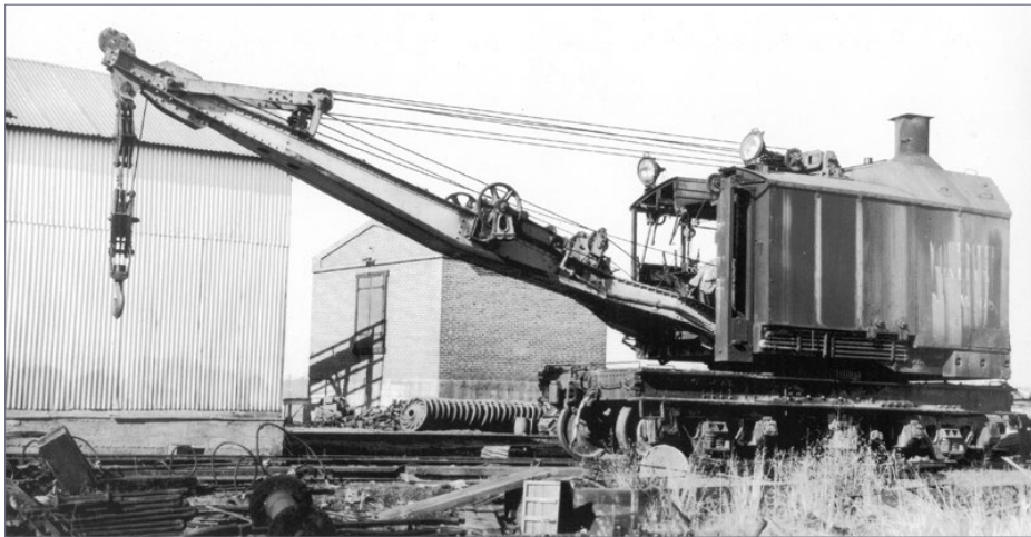
6. This photo was also taken during scrapping of the railroad. The steam crane is on a track parallel to the turntable lead and the corrugated building to the left is the sand house. This view of the oil house clearly shows both the wall toward the turntable and the blank wall along the turntable lead. Al Rose photo
