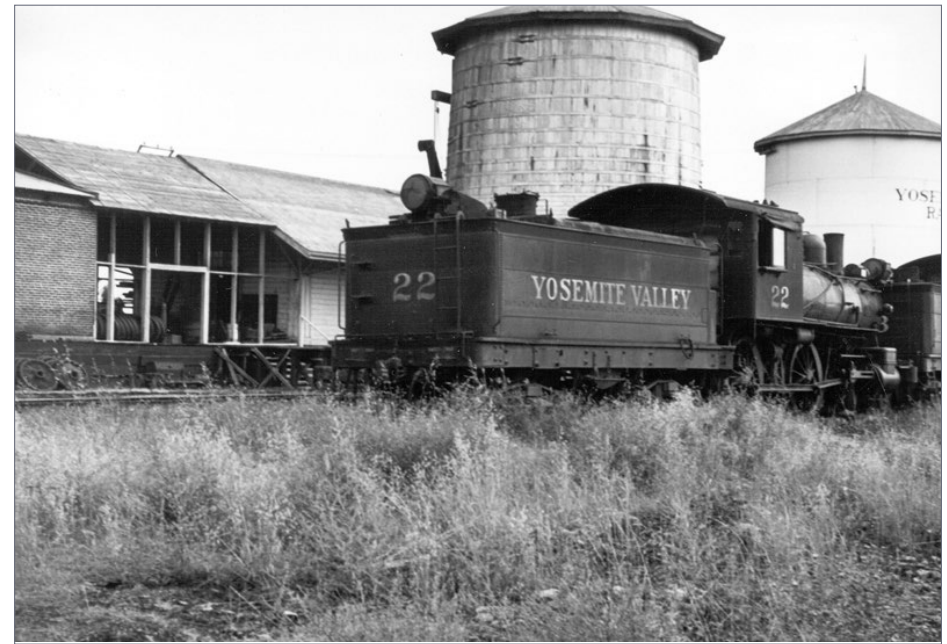
17. This photo shows the breezeway between the brick oil house on the left and the Stores building on the right. Locomotive 22 is on a track parallel to the turntable lead where the two buildings were located. Charles Givens photo
