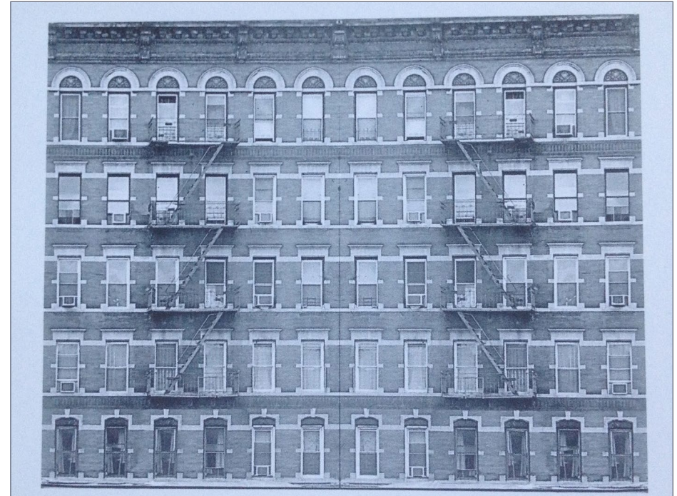
5. A copy of the building on right flipped to show different direction on fire escape.
