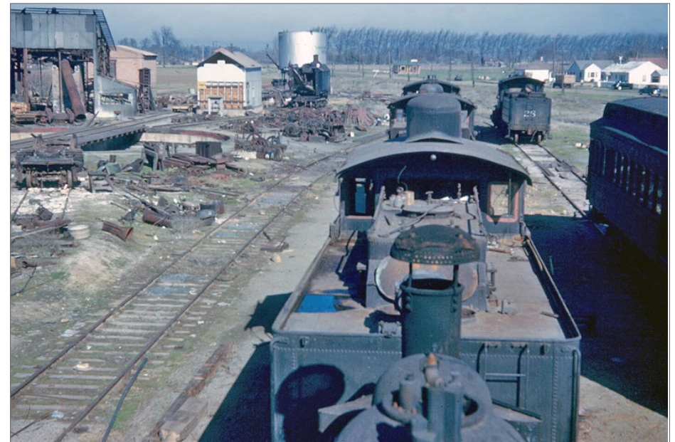
15. Al Rose stood on a locomotive to take this photo of the yards in 1946 as the railroad was being scrapped. A portion of the oil house is partly visible beyond the nearly demolished roundhouse. The shuttered window is painted black, and the brick colors are somewhat subdued. Al Rose photo
