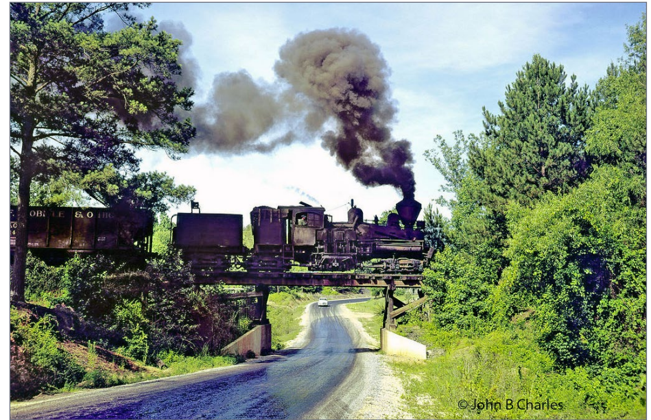
12. Shay No. 5 crossing the Kellerman "super" highway. This is the last trestle built for the extension to the new tipple. It is the only one with steel and concrete used in its construction. Photo by John B. Charles, used with permission
