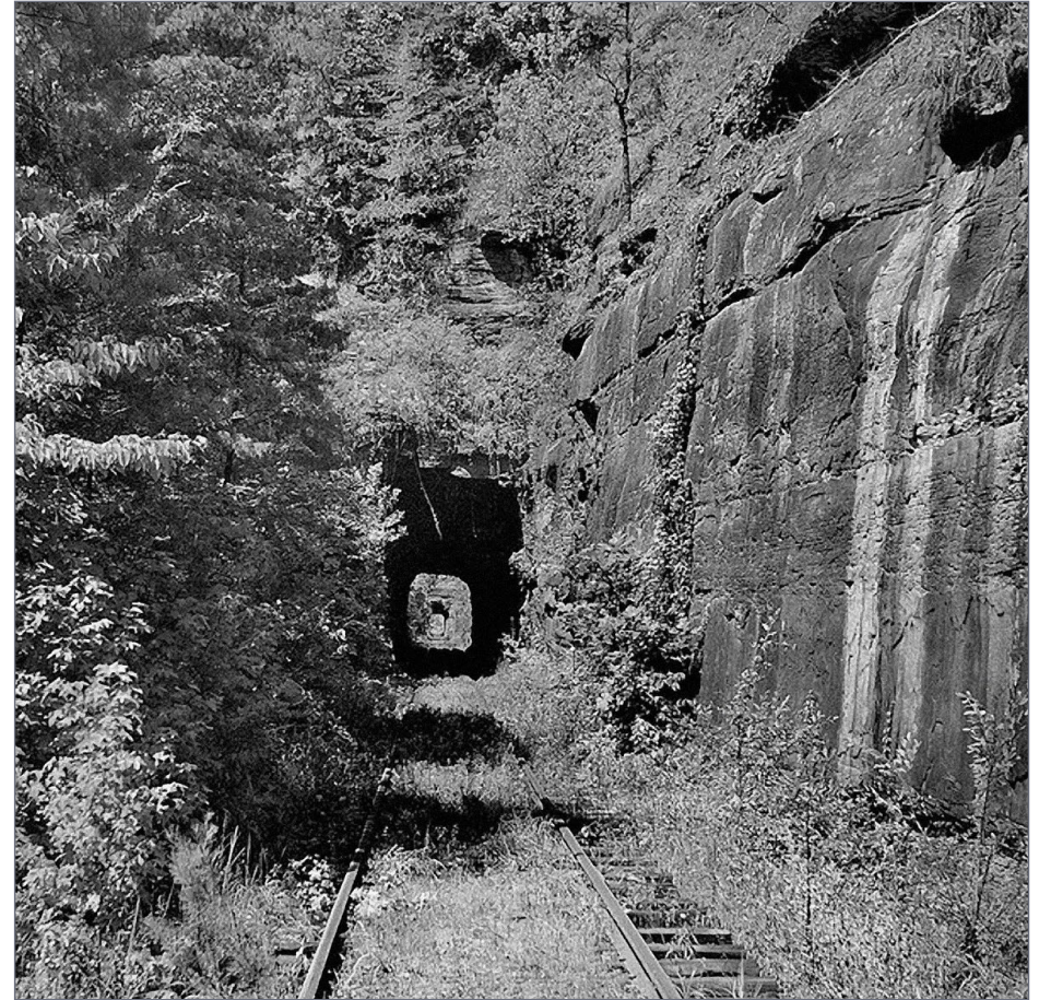
28. View is west into fourth tunnel up Daniel Creek from the Black Warrior River. The third tunnel is seen in the distance through tunnel 4 and across two trestles. Distance to the distant second tunnel portal is about 1500 feet. Tunnel 4 is 300 feet in length, then a 190 foot trestle, then through a cut and across a 225-foot trestle to 500-foot tunnel 3. William G. Gordon photo
