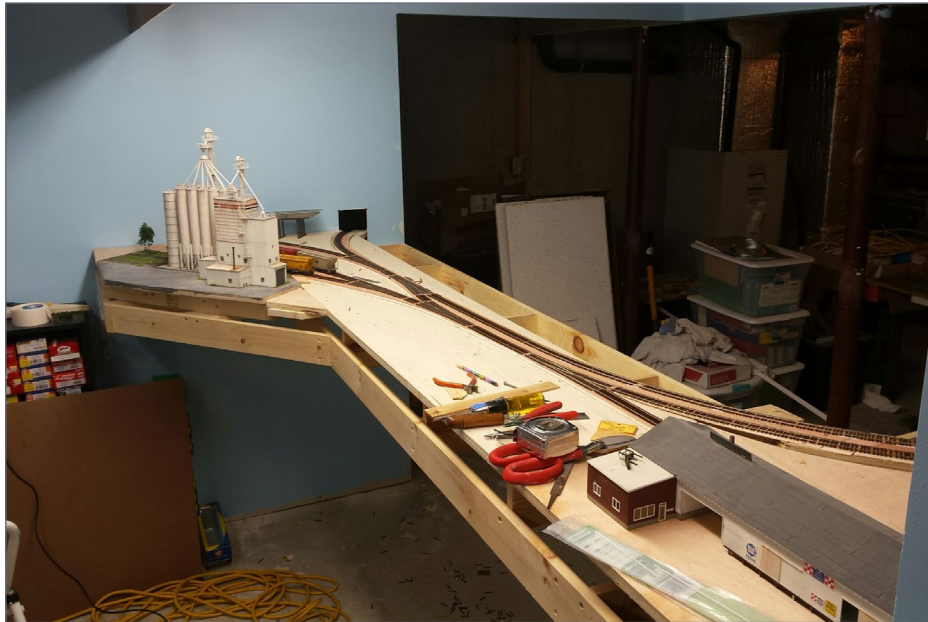
3. Completed trackwork in the Town of Bradford with primary structures placed for reference
