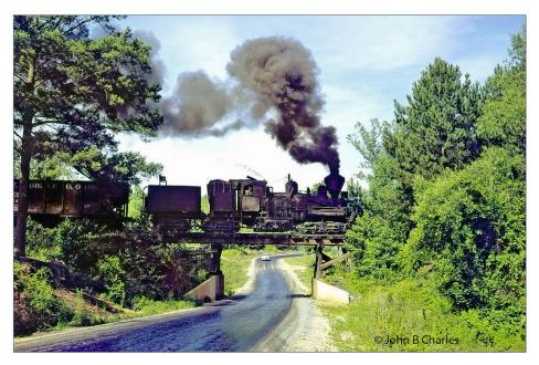
12. Shay No. 5 crossing the Kellerman "super" highway. This is the last trestle built for the extension to the new tipple. It is the only one with steel and concrete used in its construction. *Photo by John B. Charles, used with permission*
