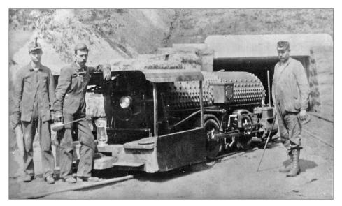
30. Compressed-air locomotive used by Twin Seam for underground operation. Central Coal and Iron 1903. Built by Porter April, 1903 C/N 2720. Photo courtesy Tom Lawson collection
