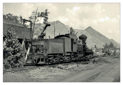
7. Shay No. 5 taking on water at the Kellerman water tank. The tank is a converted tender with a spout added. John C. Hawkins photo, <u>hawkinsrails.net</u>
