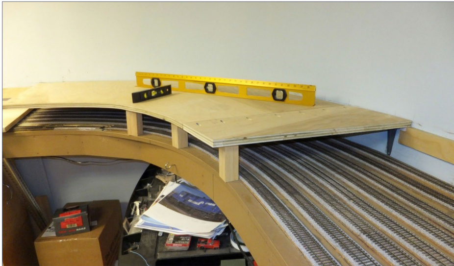
19. Wooden blocks are used as temporary supports for front of the new segment. You can't have too many levels for this kind of work.
