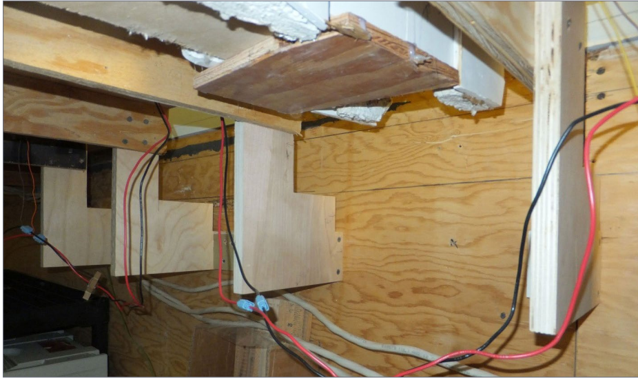
11. Viewed from underneath, you can see the "slot" created where the new pair of tracks will be installed in the cut-out of the L bracket.
