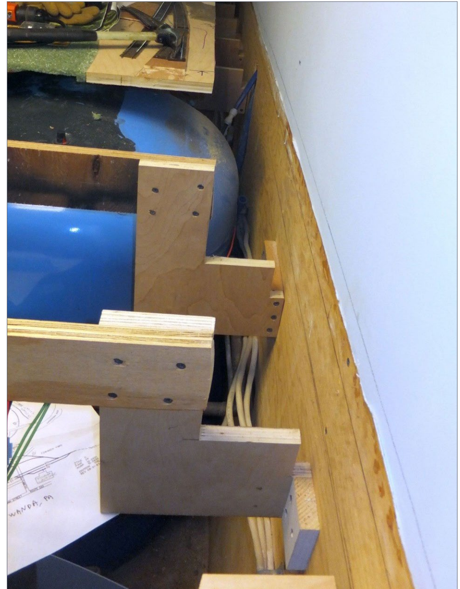
10. Looking back towards the tank and staging, you can see how the original joist ends have been cut off, and the way the new brackets now tie the benchwork to the wall.
