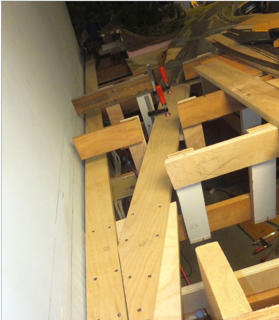
9. Looking into the original layout room and heading towards the paired hidden tracks in the "groove," you can see the new hidden tracks diverge. The left hand path will ultimately exit at Pittston Jct., while the right fork will allow the new main line to go through Towanda. Previously this was not the case, and I considered this a major improvement over the original hidden main line route.
