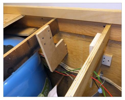
8. The pesky blue water pressure tank that has plagued many of my layout efforts was at it again! There was only one way to get two tracks to pass underneath Tunkhannock, and that was to sneak them behind the tank near the top. Clearances were tight – I just made it. The strange L-shaped plywood brackets were created so that I could chop off the existing joist ends. This was the area the new tracks needed to pass through.
