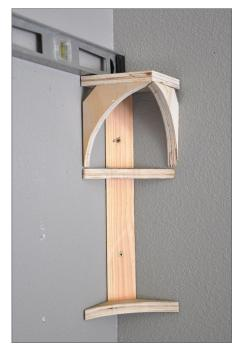
7. The corners were installed first, then I leveled the top of the backdrop using them as my height guide. The spine of the corner pieces are sections of 2x4 that I ripped at a 45° angle and attached to two of the curved pieces for the cove.
