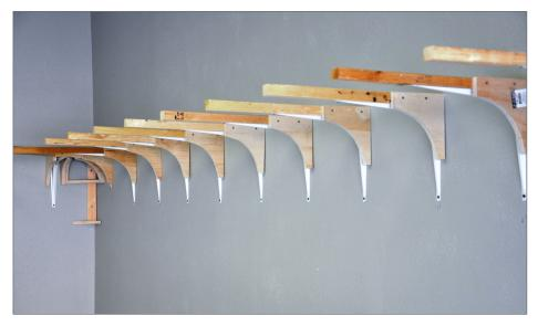
9. The shelf brackets have been installed, and 2x2 furring strips and the cove pieces have been added. Now it's time for the Masonite.
