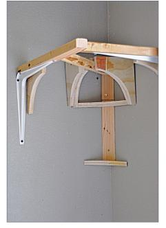
8. I added the brackets and extensions adjacent to the corner pieces, plus some additional cove pieces so there is plenty of material to screw the Masonite into.
