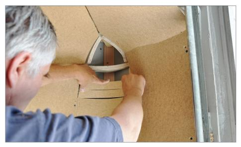
11. I filled in the corners with small pieces of Masonite, test-fitting each piece before I nailed it in place.
