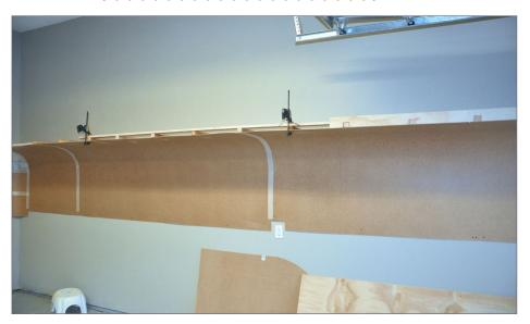
15. After all of the Masonite was installed, I attached a piece of 1 furring strip across the top of the backdrop. I added a 4" strip of plywood across the top to anchor the front face of the backdrop. I used my table saw with a dado blade to notch out for the 2x2.
