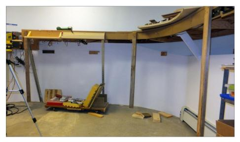
13. How do you lower a 22-foot-long curved staging yard? You do it very carefully and with a lot of planning. Shown here are temporary legs screwed to the front of the existing yard benchwork, along with cleats on the wall where the rear of the bench work will rest until screwed to the studs.
