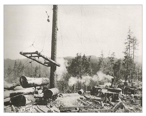
3. At the loading site, a large central "spar tree" was cleaned and rigged with boom, pulley blocks and lines to position cut logs on rail cars. Steam donkeys reeled or released the various lines to swing, raise, and lower the boom. Donkey engines also were used to pull logs from cut locations to the loading area. Gravity was often used to roll the empty flat cars into place below the boom. Note the tong hooks which grip into the logs.
