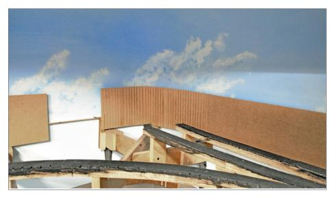
29. I added the Masonite spacer between the backdrop and where the foam scenery base will be. This keeps the rest of the scenery separated from the sky.
