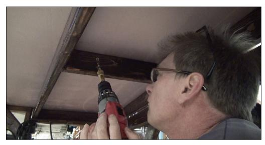
16. To prevent the foam from sliding on top of the bench work when pushed or bumped, I drill countersunk holes in to the bottom of the wood, and drill three-inch screws up into the foam. This holds it firm yet makes it easy to detach quickly to move the layout outside for photos or video when needed.
