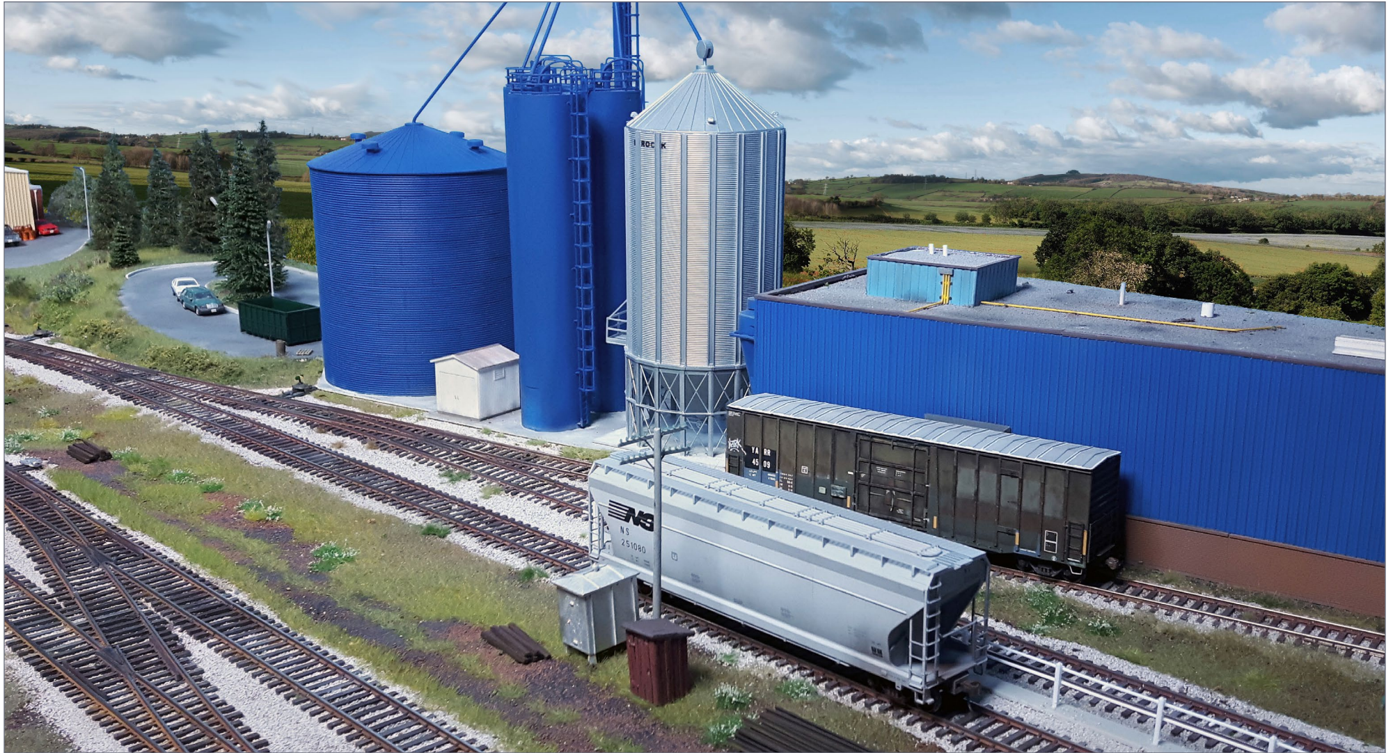
19. The finished kitty litter plant scene.
