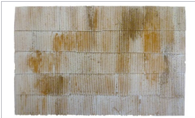
49. Completed corrugated siding.
