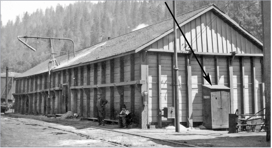
23. The south end of the SP sand house at Dunsmuir had a fire equipment cabinet, indicated by the arrow, and it was painted bright red. Notice it is supported off the ground. This is the type of cabinet I decided to model. SP photo, Shasta Division Archives, courtesy Bob Church
