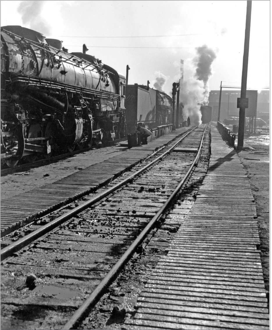
5. This photo of the wash rack north of the roundhouse at SP's Taylor Yard in Los Angeles, taken in the summer of 1950, shows the duckboards provided so workmen's feet could mostly stay out of the accumulated oil and water in the area. Richard Steinheimer photo, DeGolyer Library
