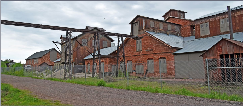
10. The Quincy Smelter in Hancock, Michigan.
