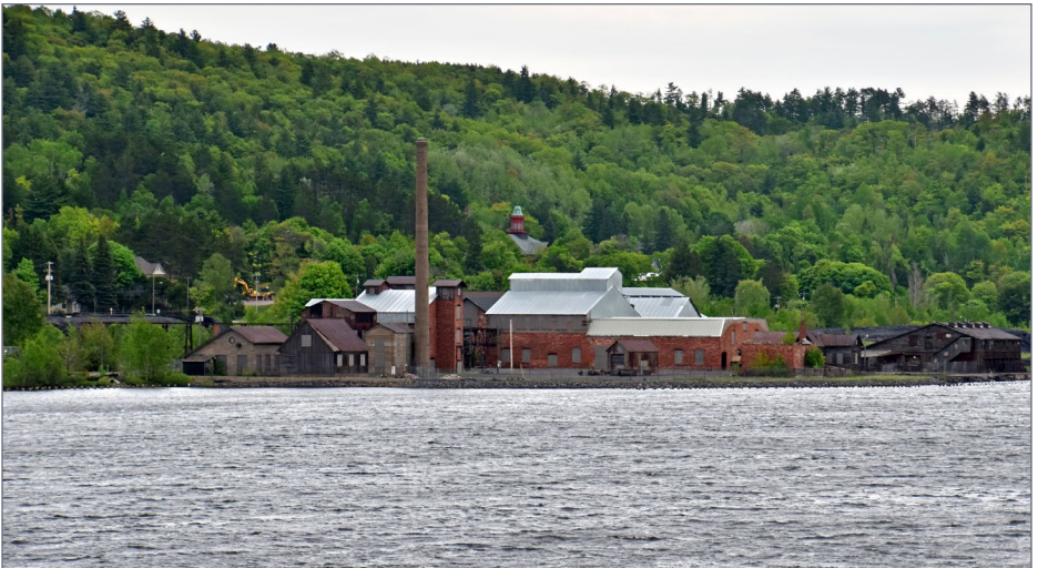
11. The Quincy Smelter as viewed from the Portage Canal lift bridge.
