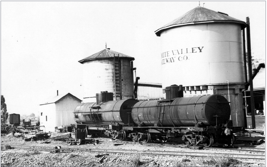
18. A pair of tank cars on the track along the back side of the oil tank. The nearest car is spotted over the drain connection. Ted Wurm photo
