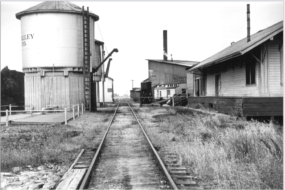
11. Looking down the turntable lead track toward the roundhouse. On the left is the oil settling tank, oil tank, water tank, and sand dryer house. On the right is the stores building, oil house, and a storage building made from retired combine 105. Charles Givens photo
