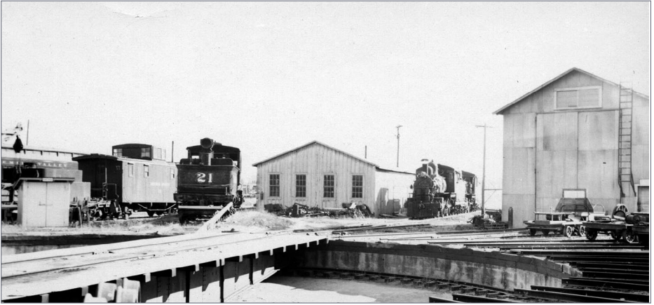
26. This view from the turntable (the roundhouse is out of view on the right) shows the prototype paint shop, the wood-working shop and, on the left, the fire hose shed. Fred Stoes photo
