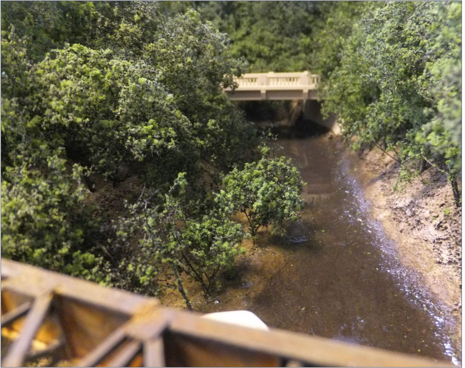
58. A view “standing” on the ballasted track portion of the rail bridge, with the Route 6 road bridge in the distance.
