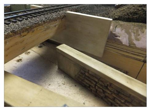
42. There was actually leftover spline sub-roadbed in this area, but it proved ideal for it to simply continue and build the bridge around it, since it was a ballasted deck. Here I'm fitting the New England Brownstone rear retaining casting around the sub-roadbed spline. I find it very easy to accurately cut the castings on my band saw.
