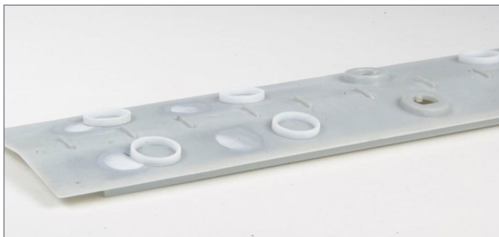
8. New roof hatch bases glued in place.
