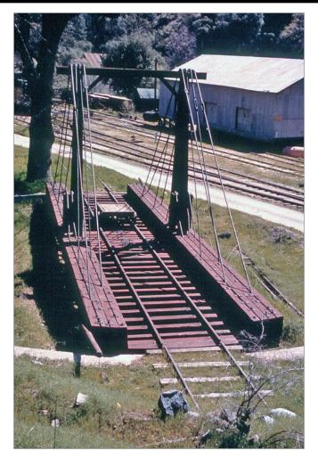
6. Looking down on the turntable with its short extension track. This turntable was used only to turn locomotives and passenger cars (such as the observation car). The approach track is overgrown with grass, and the road crossing covers the rails, confirming that the turntable wasn't being used by the time of the photo. The Government Warehouse is on the other side of the tracks. Note the pair of rails half-buried in the turntable pit. *Al Rose photo*
