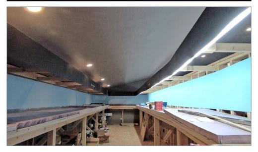
26. The benchwork is built from 2x6 and 2x4 board with a rail height around 54". With backdrops painted blue, and valance lighting all the way around the layout, it is time to start laying track. Look forward to updates on "What's Neat," as progress continues on this magnificent home layout project.
