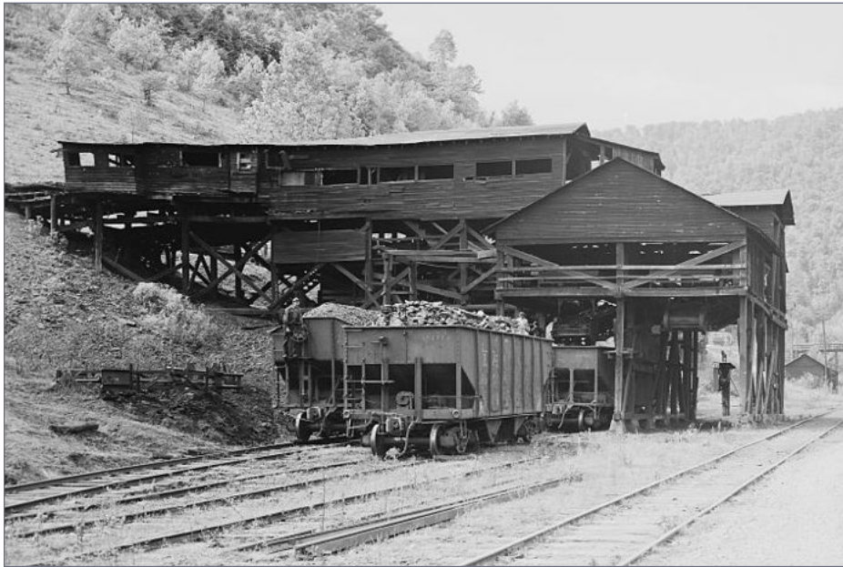
10. Example of a coal loader suitable for modeling. This building could be connected to a mineshaft, but it's equally possible it is connected to a conveyor belt or a truck dump. There is probably a space for sorting and grading coal in the structure, with different sizes loaded on different tracks. This mine was part of the PV&K coal company in eastern Kentucky.
