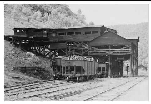
10. Example of a coal loader suitable for modeling. This building could be connected to a mineshaft, but it's equally possible it is connected to a conveyor belt or a truck dump. There is probably a space for sorting and grading coal in the structure, with different sizes loaded on different tracks. This mine was part of the PV&K coal company in eastern Kentucky.
