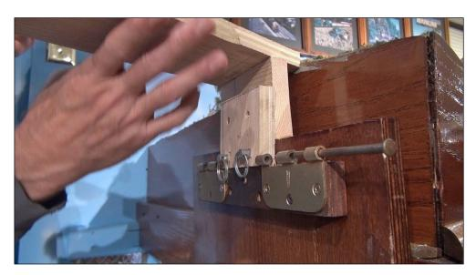
7. These pins fit through the holes, making for a very solid attachment point to the existing stained <sup>3</sup>/<sub>4</sub>-inch plywood fitting between the old door hinges. The pins easily pull out with the help of a metal ring pull that your finger fits into.
