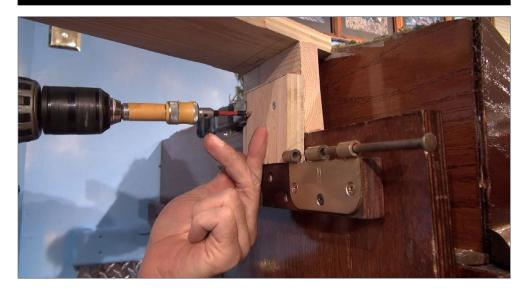
5. I used wood screws to join the lap joint and attach the <sup>3</sup>/<sub>4</sub>-inch plywood to the 1x4 riser. I then drilled two 3/8-inch diameter holes in the 1x4 and the existing stained plywood, about 3 inches apart.
