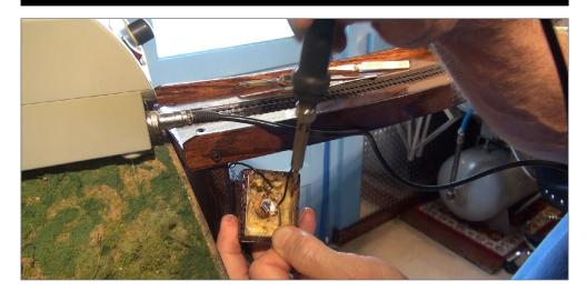
12. I drilled two holes in the lift-out section to run power wires from the rails through the <sup>3</sup>/<sub>4</sub>-inch plywood, feeding the wires into the small wood box and soldering the leads to the microphone jack solder tabs.
