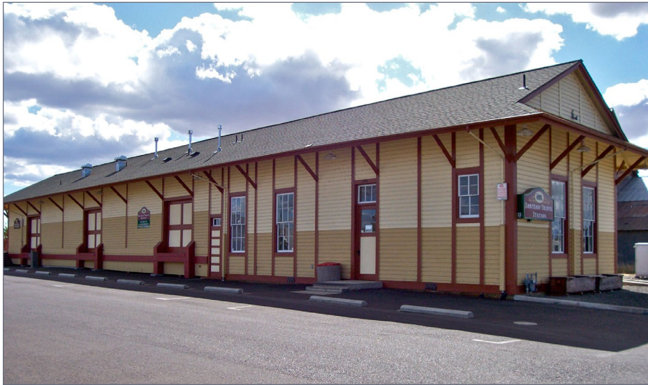
12. Restored Southern Pacific train station in Lebanon. Source: Wikipedia
