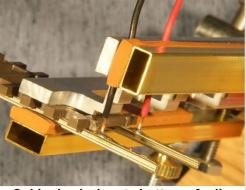
Solder lead wires to bottom of rails
