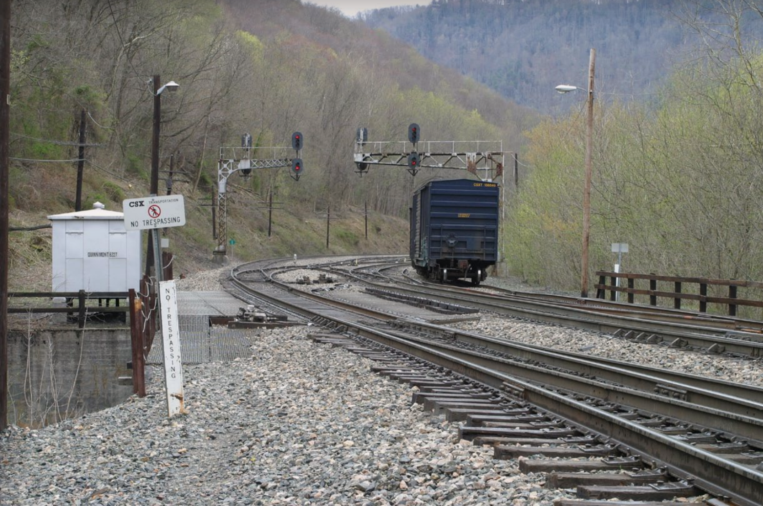
FIGURE 4: Modern mainlines with today's ▲ heavier cars typically use 130 to 135 pound-per-foot rail that's just over 7 inches high. In N scale, that equates to approximately 45 thousands of an inch, or code 45 rail.
