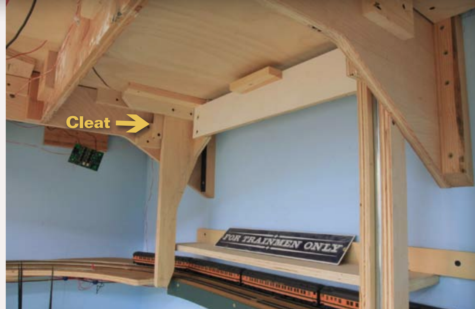
FIGURE 9: A view under the lowered hatch. Be sure to allow space for those drawer slide assemblies - they project downward 18"! Deschutes staging (2 tracks) is under the hatch necessitating the shelf above as protection from errant elbows and hips. Note the position of the disengaged locking cleat allowing the drawer slide assembly to move past it.
