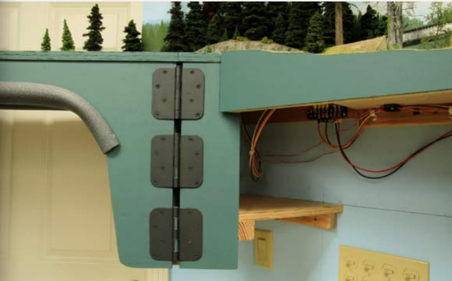
FIGURE 18: A movable bridge with track on it requires secure abutments. I used 'box' style construction to build mine. Note the three hinges. They need to be good quality because they set the horizontal alignment at the hinge end. If they get sloppy the tracks won't line up right. The axis the gate pivots on should be absolutely vertical.
