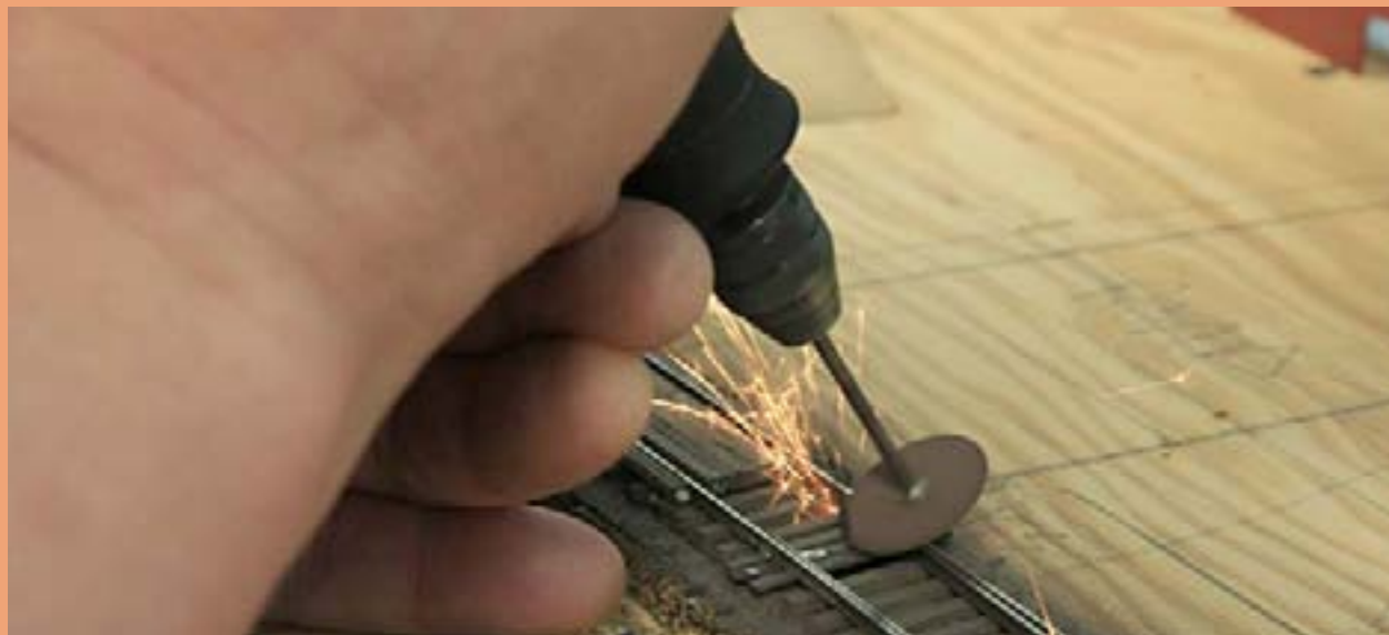
Figure 44: Trimming the actuator wire above the throwbar.
