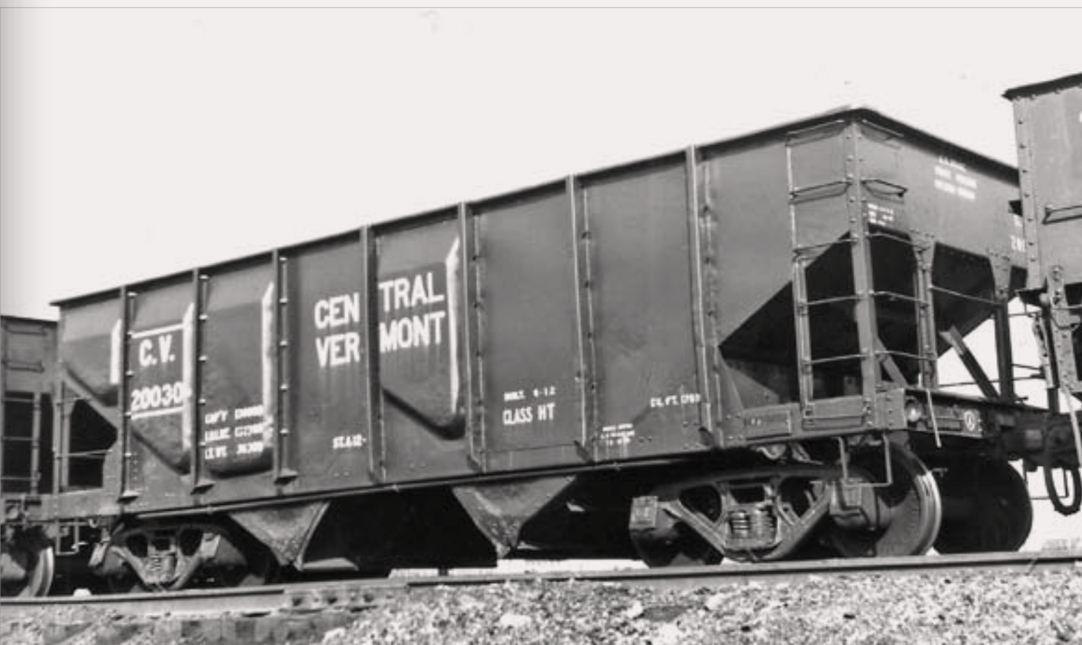
Figure 5 & 5a: The Central Vermont owned 200 steel hopper cars, built in 1912 and numbered 20000-20199, which were slightly smaller than the USRA hoppers. Starting in the mid-1930s, these cars were rebuilt with panel sides, new AAR cast steel trucks, and geared hand brakes. CV 20005 was photographed fresh from the St. Albans, VT shops after being rebuilt in January, 1937. Not all of the CV hoppers got complete sets of panel sides; when photographed in the early 1940s, CV 20030 had only four replacement panel sections. –Both, author’s collection
