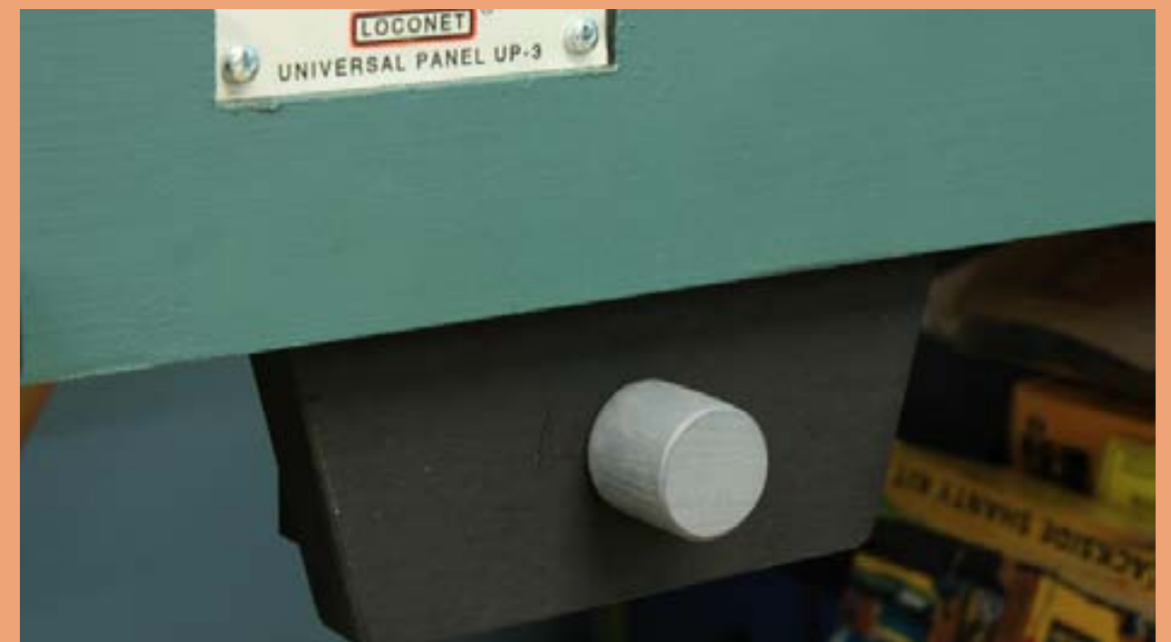
Figure 24: Turnout control installed below fascia.
