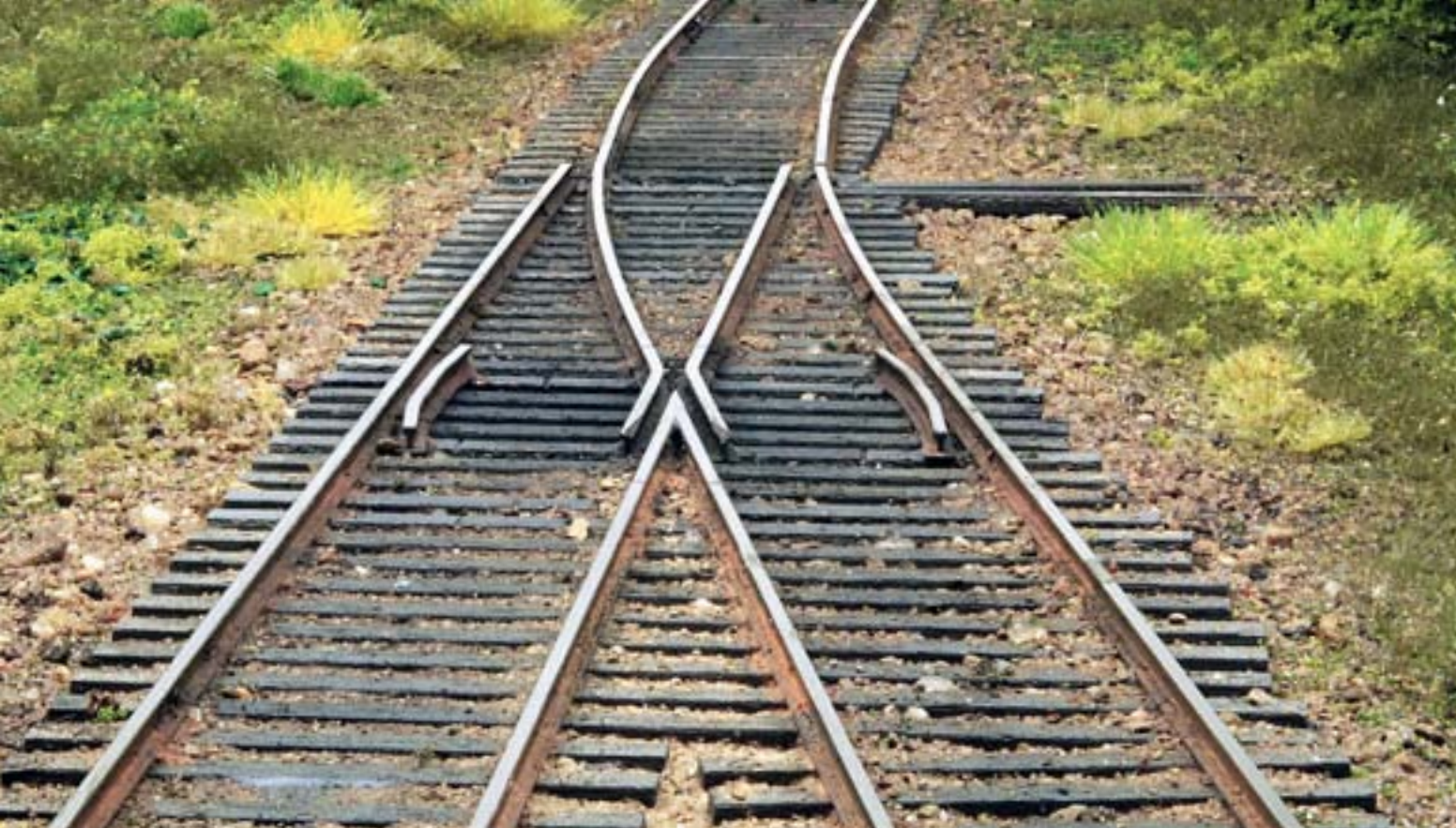
FIGURE 8: Completed stub turnout, painted, ballasted and scenicked in place.
