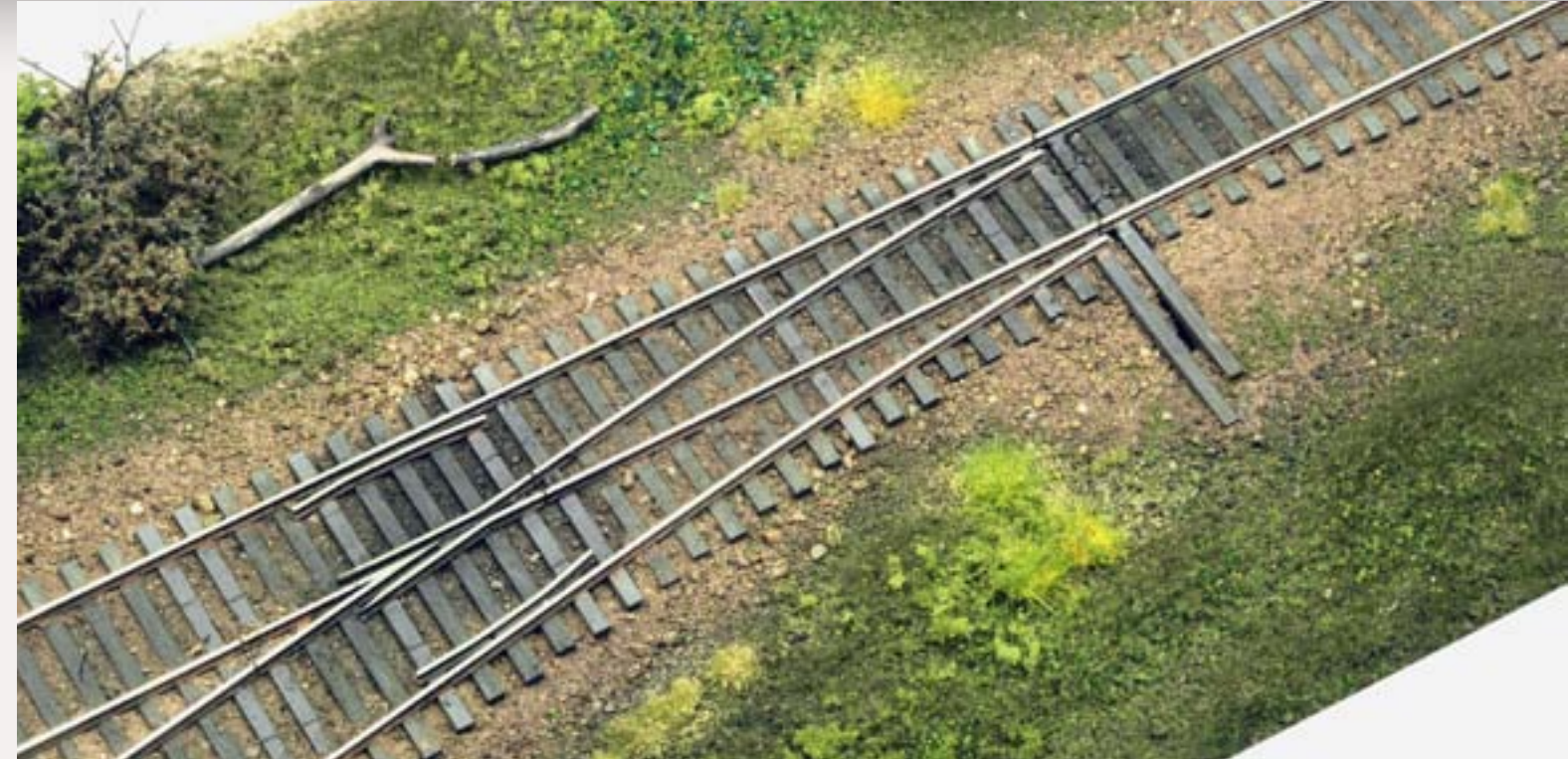
FIGURE 6: The “switch” portion of a stub switch is the same as a modern turnout, missing are the moveable switchpoints, instead a moveable bridle was used.
