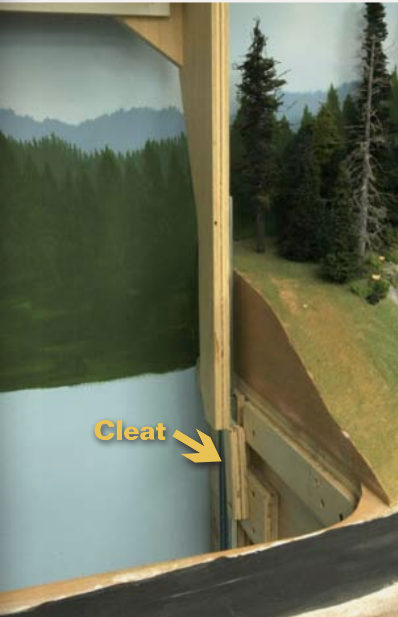
FIGURE 3: The right hand support leg of the hatch. Note the 'cleat' under the hatch 'leg' holding it in the 'up' position.
