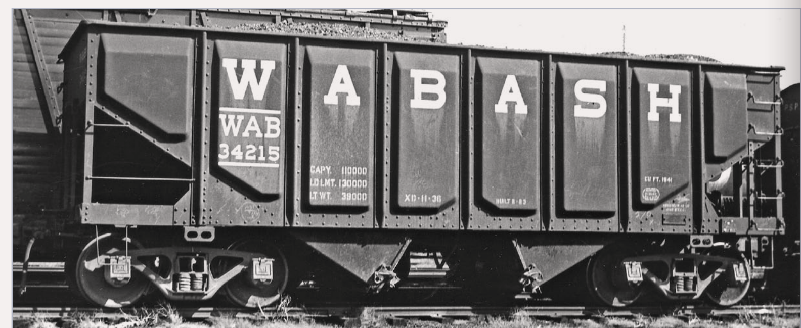
Figure 7: The Wabash received 1000 twin hoppers from the USRA and then purchased additional cars of similar design in the early 1920s. The Wabash was so enthusiastic about replacement panel sides for its twin hopper cars that it not only rebuilt almost all of them as panel side cars in the 1930s but, beginning in 1937, constructed almost 2000 new panel side hoppers in its own Decatur, IL shops. WAB 34215, originally one of 750 31000-31749 series USRA-design cars built in 1923, is shown here at East St. Louis, IL in 1938 after being rebuilt with panel sides at Decatur in November, 1937 and renumbered into the 34000-34499 series. –Joe Collias collection.
