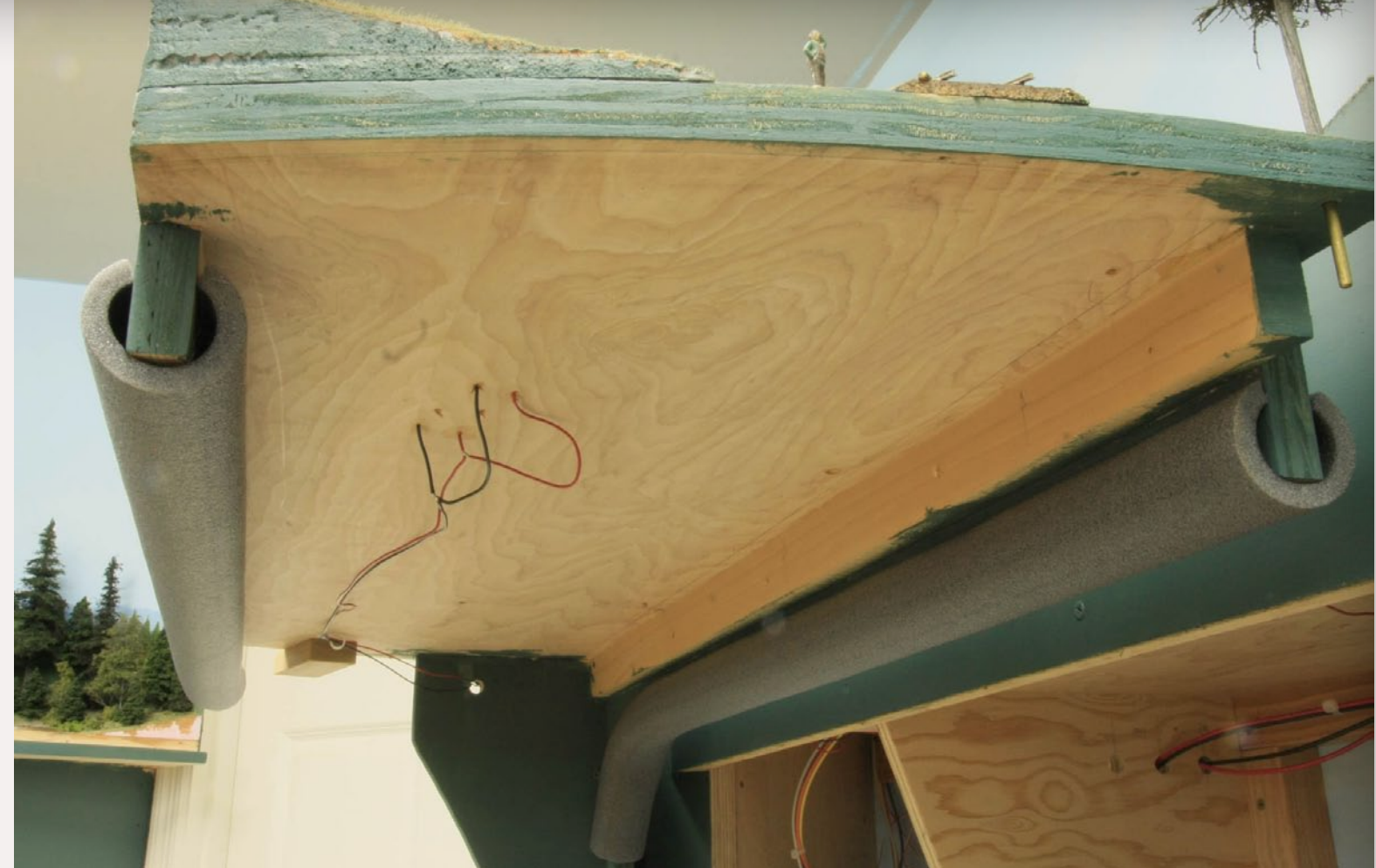
FIGURE 19: I ran 'ribs' down the front and back of the bridge to avoid sagging. These got covered with grey foam pipe insulation (to protect heads!). Note the locking pin with the tree on top at the far right.
