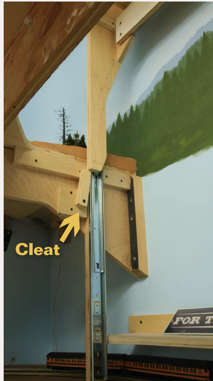
FIGURE 4: An extended drawer slide is clearly visible here as is a 'cleat' holding up the hatch 'leg'. The cleat pivots around the single screw attaching it.
