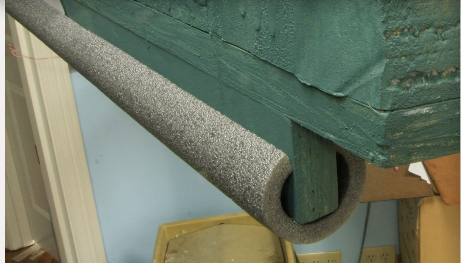
FIGURE 14: Plumbing insulation foam makes good head protection for early risers.
