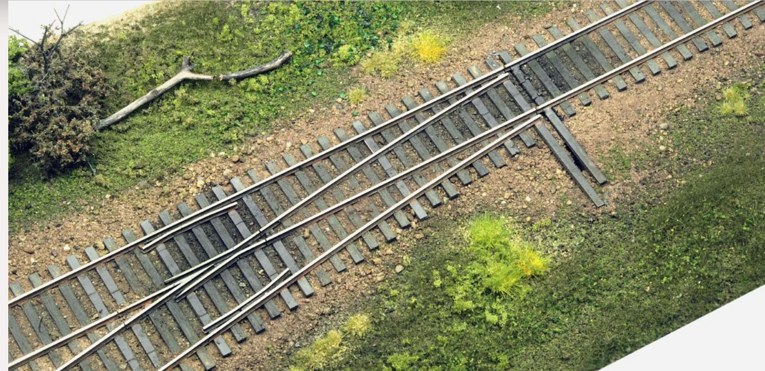
FIGURE 6: The “switch” portion of a stub switch is the same as a modern turnout, missing are the moveable switchpoints, instead a moveable bridle was used.
