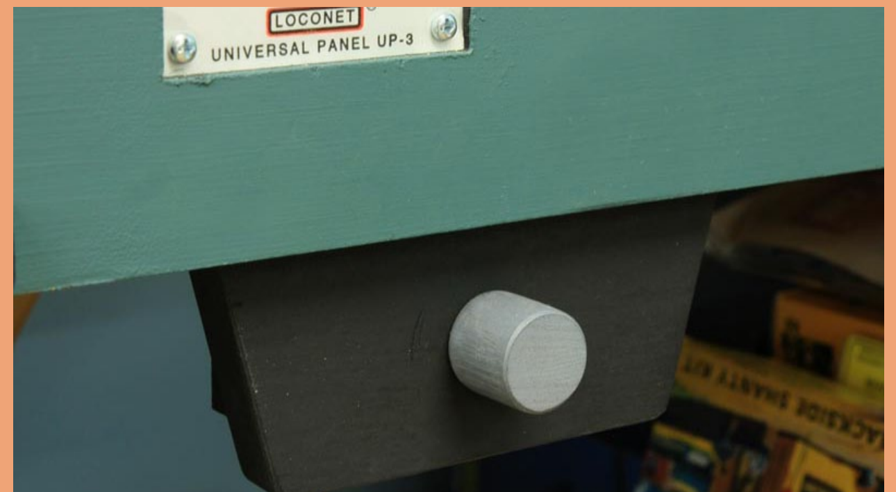
Figure 24: Turnout control installed below fascia.
