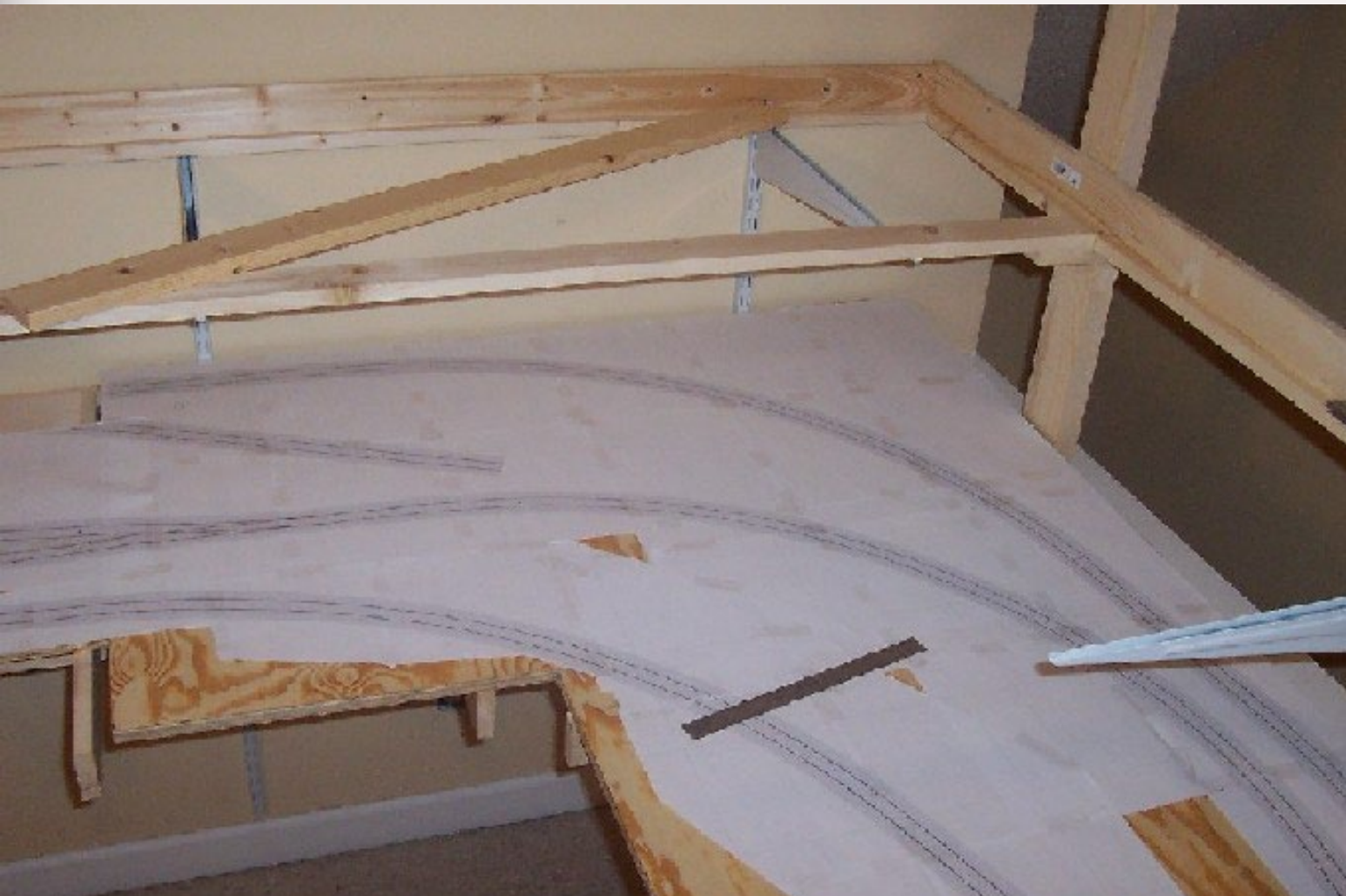
Figure 28: I make cuts every 6 inches down the centerline.
