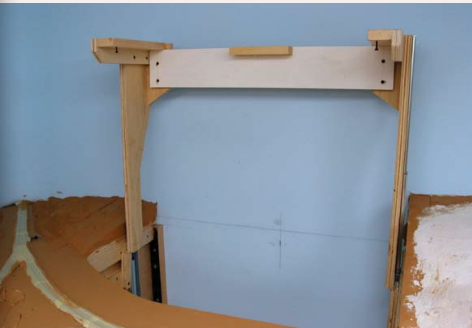
FIGURE 8: The hatch supports with the hatch top removed. Note the bracing at the top which helps keep this assembly relatively stiff.
