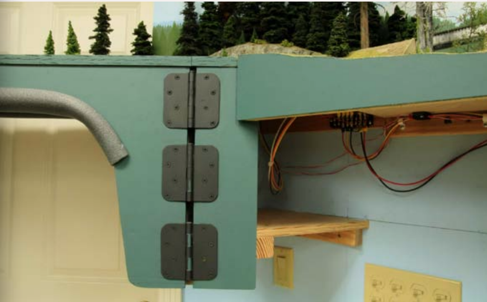
FIGURE 18: A movable bridge with track on it requires secure abutments. I used 'box' style construction to build mine. Note the three hinges. They need to be good quality because they set the horizontal alignment at the hinge end. If they get sloppy the tracks won't line up right. The axis the gate pivots on should be absolutely vertical.
