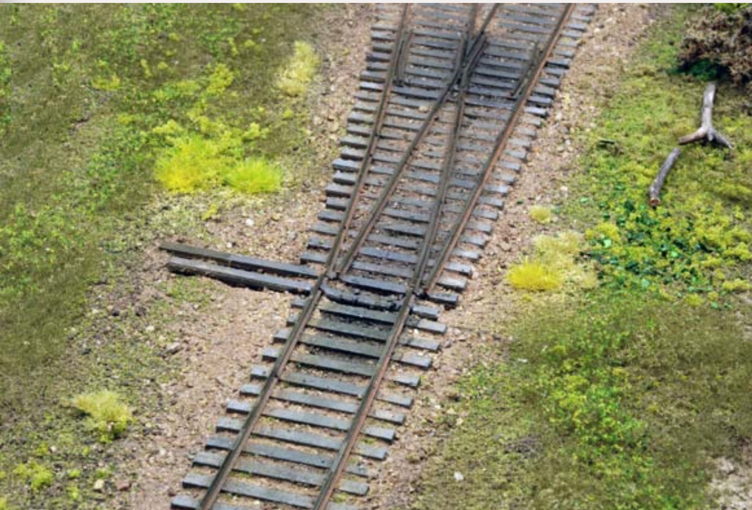
FIGURE 2: Stub switches, once common at the turn of the century, are now relegated to museums and tourist railroads.
