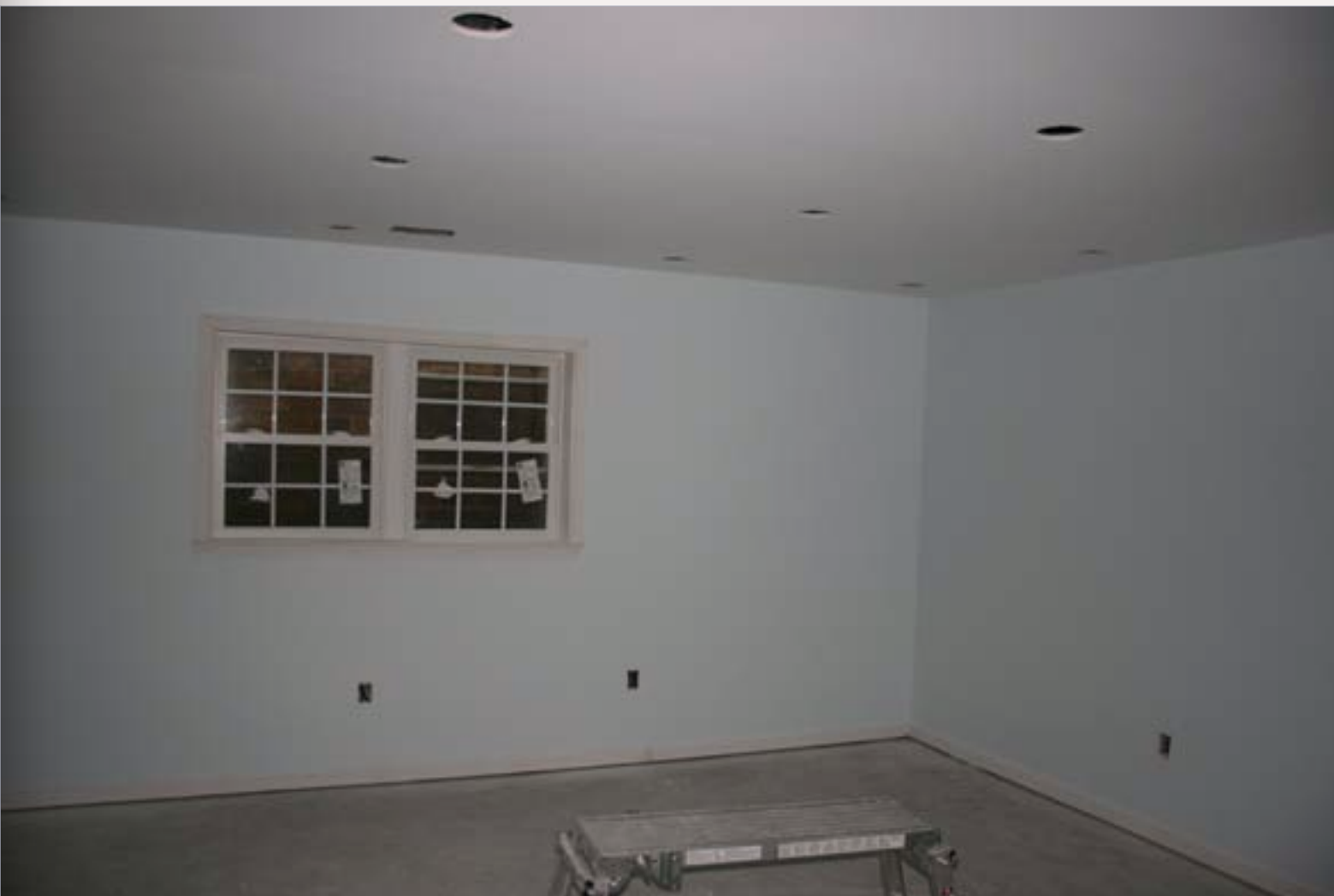
FIGURE 1: Nice new basement to fill full of layout!!
