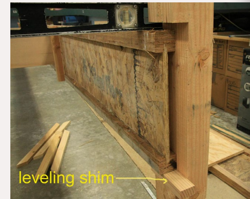
FIGURE 15: Shimming the engineered joists to level them.
