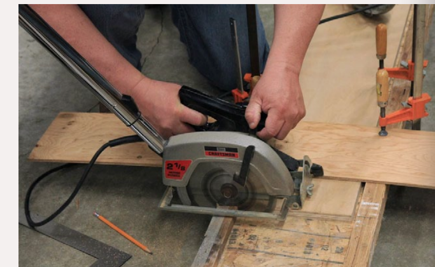
FIGURE 14: cutting the engineered beams to length. Using the vacuum keeps dust generation to a minimum in the train room.
