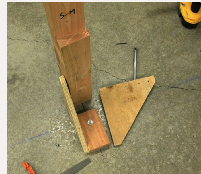
FIGURE 13: Installing a 4x4 leg for the peninsula using a concrete anchor to fasten it to the floor.
