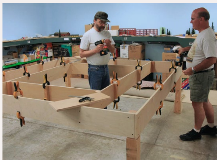
FIGURE 10: Construction of the helix table under-the-surface bracing.
