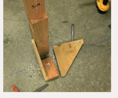
FIGURE 13: Installing a 4x4 leg for the peninsula using a concrete anchor to fasten it to the floor.
