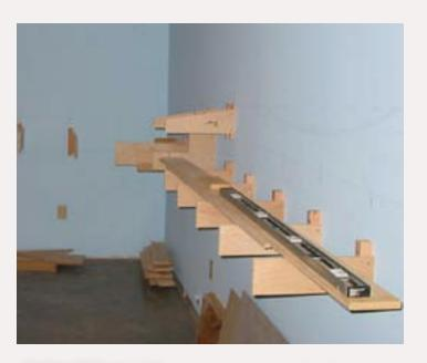
FIGURE 5: More joists and cleats.
