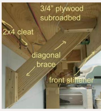
FIGURE 2: Under Mill Bend.
