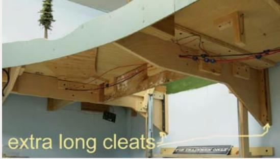
FIGURE 7: Long joists below Oakhill with extra long cleats extending downward.
