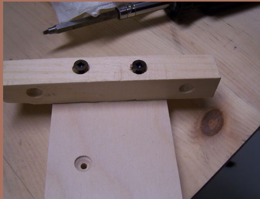
Figure 24: Adding a cleat to the top of each riser.
