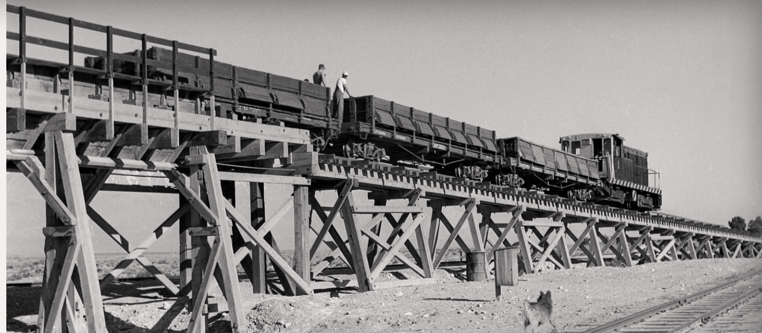
Figure 14: SP narrow gauge GE #1 works the ore trestle at Owneyo in 1955. The side-dump gondolas had an internal "A-frame" pitched floor to facilitate dumping into standard-gauge cars below. This view illustrates well the actual configuration of the high-line trestle. The layout compromises by having the standard gauge duck down because the narrow gauge can't climb enough in the space available. Looks like crews might have re-laid the narrow gauge track in the foreground (headed to Keeler) with some standard gauge ties. Courtesy, Joe Dale Morris Collection.
