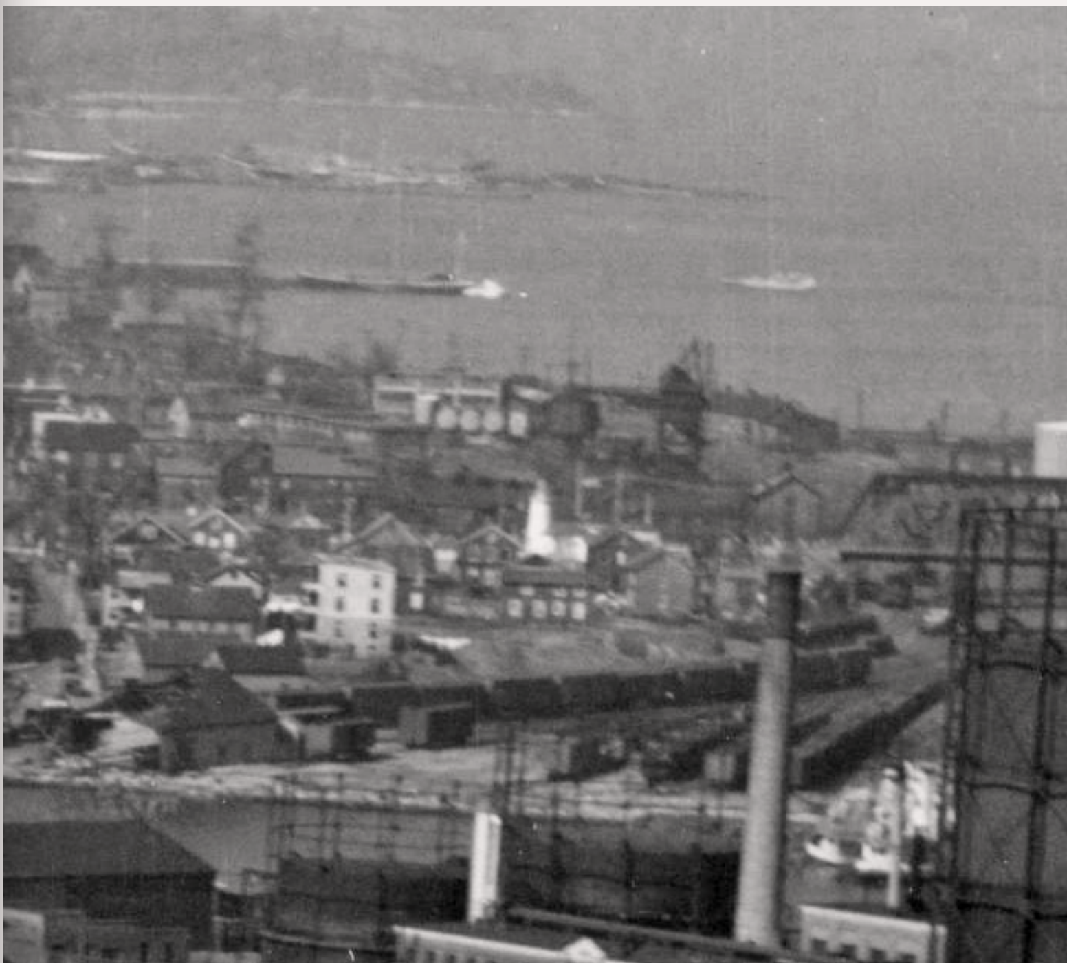
FIGURE 12: The CV coaling tower can be seen in this image. Bulk oil distributorships (which received oil in barges, stored it in tanks, and then shipped it either to local customers by truck or further distances by rail) were common in New England coastal towns through the 1960's. An oil tank of one such distributor can be seen in the extreme right edge of this photo.
