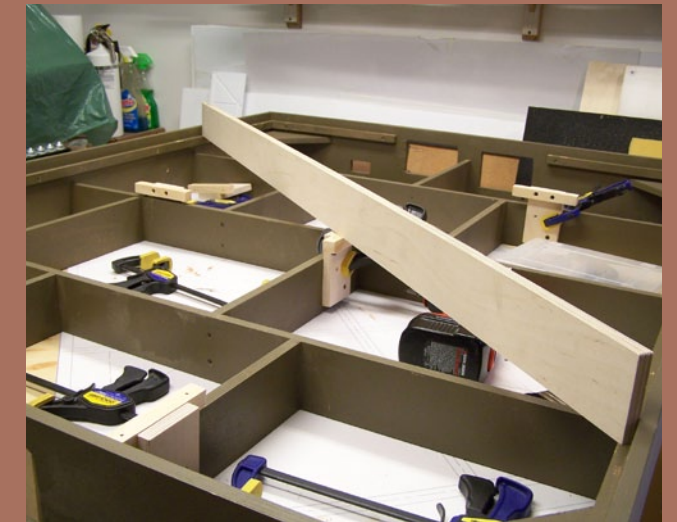
Figure 29: Installing and levelling the risers.
